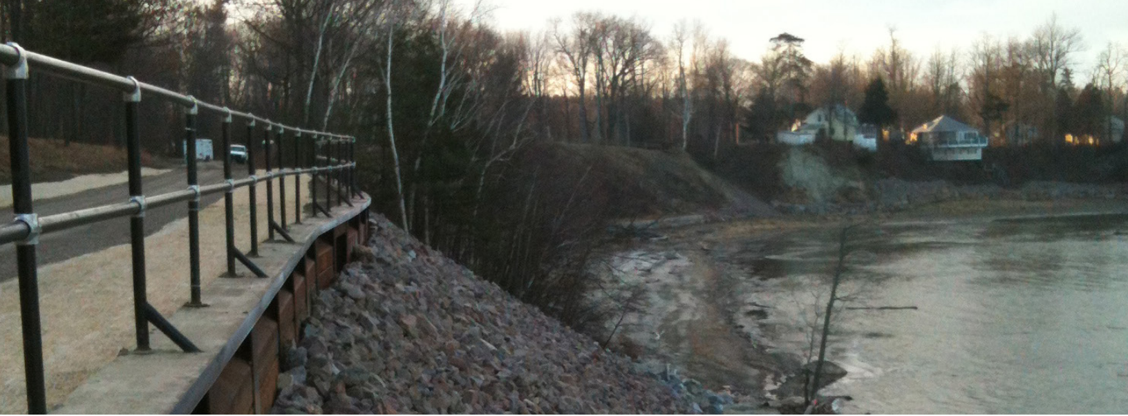
Burlington Bike Path Slope Repair, Burlington, Vermont
