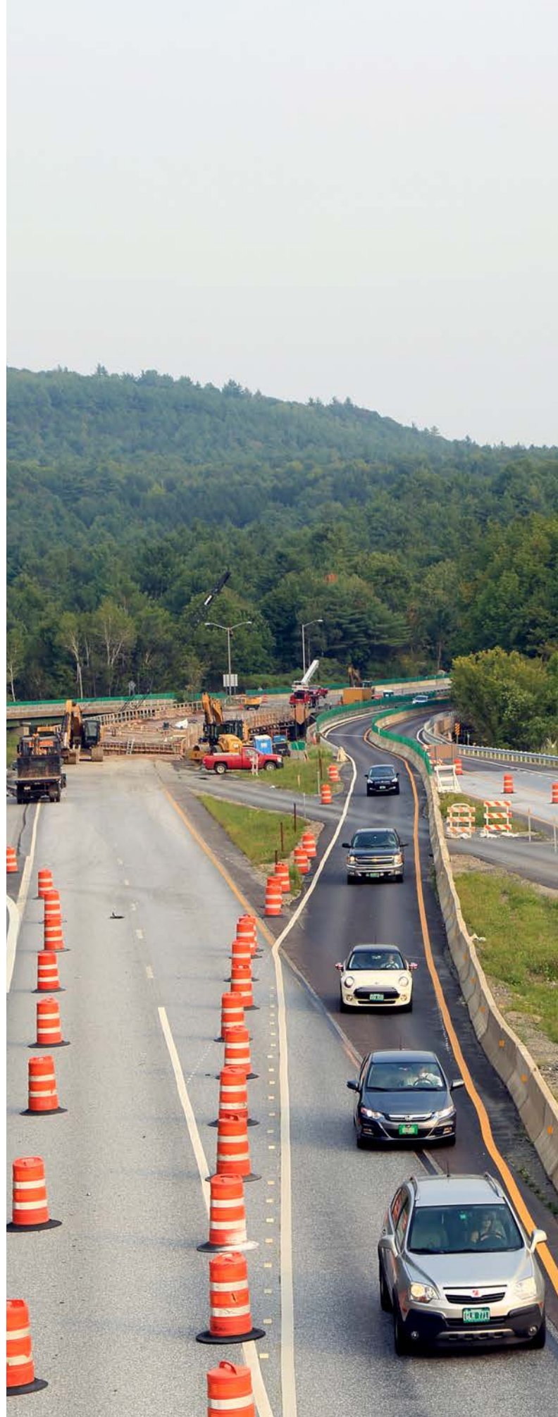
Waterbury I-89 Exit 10 Bridge, Waterbury, Vermont
