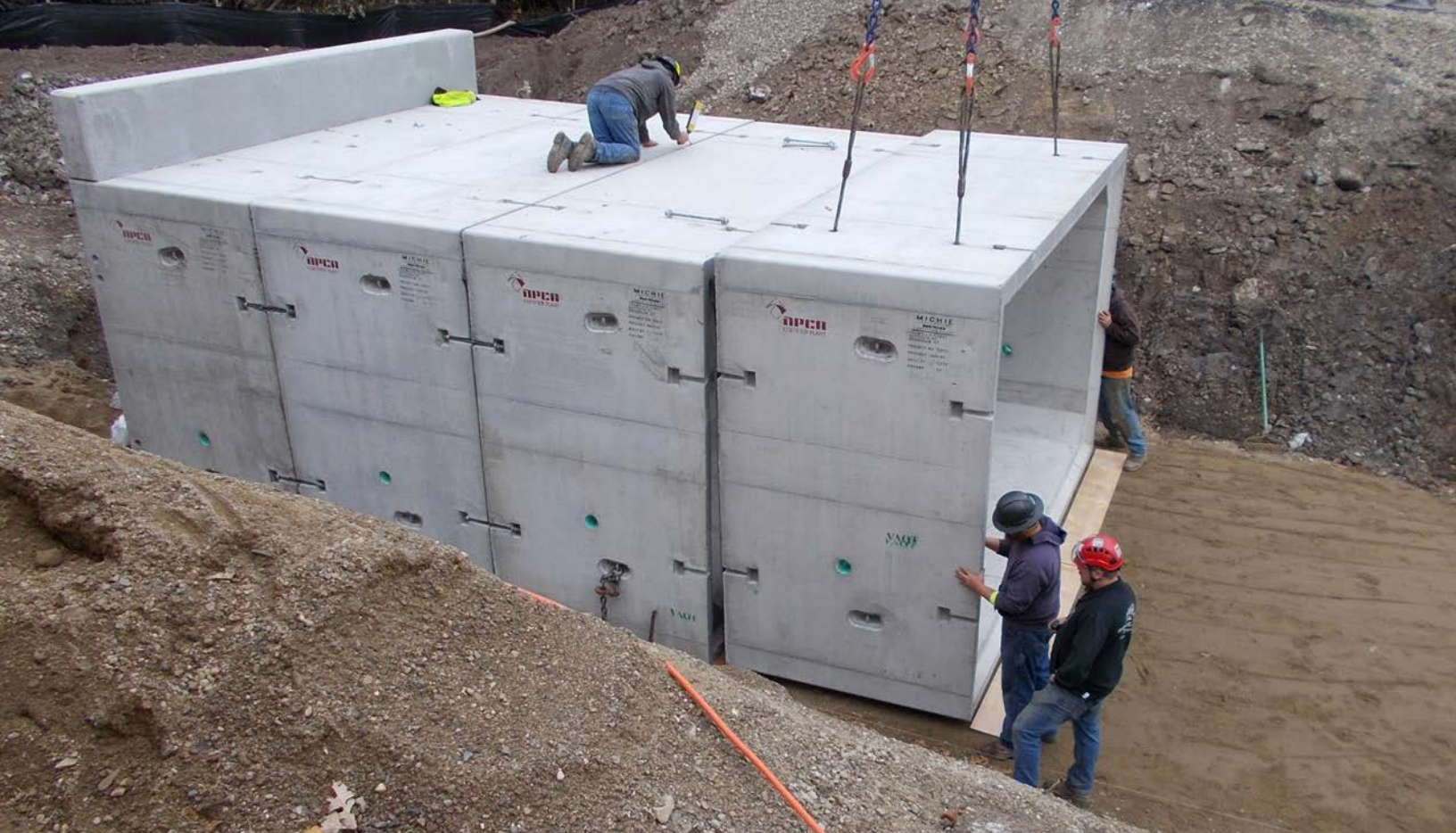
Shoreham Buttolph Road Culvert, Shoreham, Vermont
