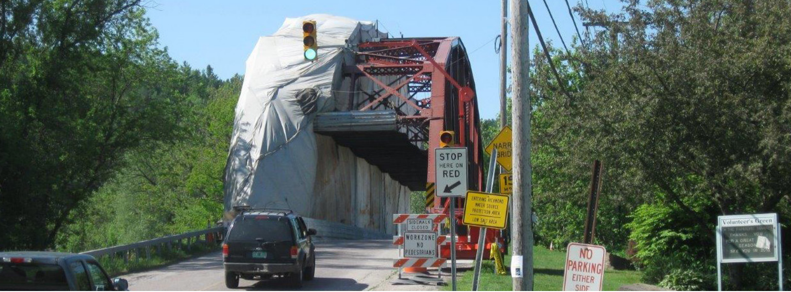
Richmond Bridge Painting, Richmond, Vermont
