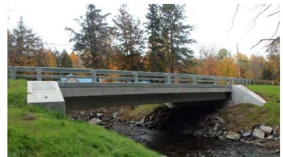
Bridge Replacement in Barton Fuss & O'Neill performed a complicated replacement of a 26-foot span concrete T-beam bridge over Roaring Brook in Barton. The project went through the VTrans Municipal Assistance Section process. Many improvements were made while staying within the existing Right-of-Way. The bridge was part of the Accelerated Bridge Program and was closed for four weeks for construction.
