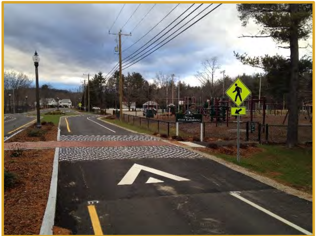
Union Street Roadway Reconstruction, Pedestrian Facilities, Stormwater, Sewer Replacement, Lighting Peterborough, New Hampshire
