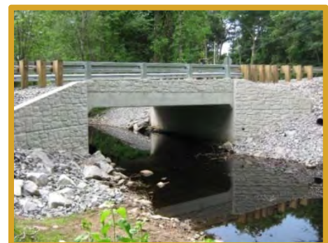
Drew Road Culvert Replacement Derry, New Hampshire
