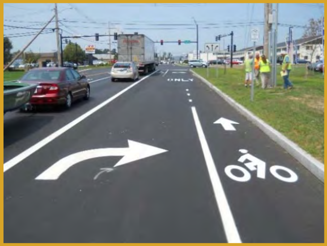
Manchester Street/Airport Road Intersection Reconfiguration & Signalization Concord, New Hampshire
