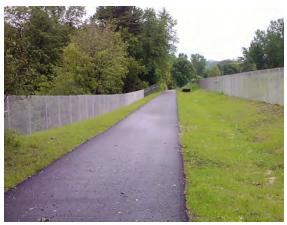
Route 127 Recreation Path Restoration Fuss & O'Neill repaired and replaced an eight foot wide section of the recreation path that suffered slope failure. The project involved removal of the failed pavement and subbase, and replacement and restoration in-kind with extruded polystyrene block as lightweight backfill.
