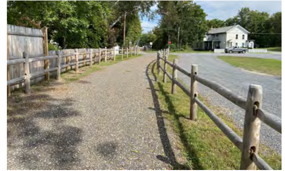
Delaware and Hudson Rail Trail Fuss & O'Neill provided upgrades that included grading and resurfacing the nearly 20-mile Delaware and Hudson Rail Trail that extends over two sections across southwestern Vermont.
