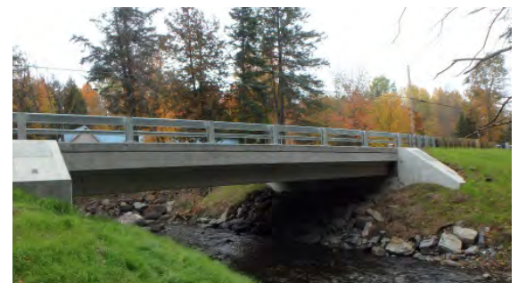
Bridge Replacement in Barton Fuss & O'Neill performed a complicated replacement of a 26-foot span concrete T-beam bridge over Roaring Brook in Barton. The project went through the VTrans Municipal Assistance Section process. Many improvements were made while staying within the existing Right-of-Way. The bridge was part of the Accelerated Bridge Program and was closed for four weeks for construction.
