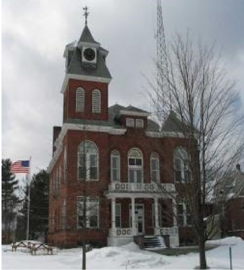
Lamoille County Courthouse
