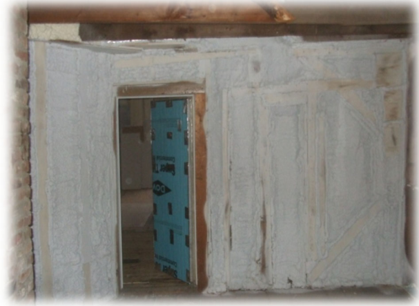
Above, spray foam was utilized to separate an unheated storage area from the rest of the home.
