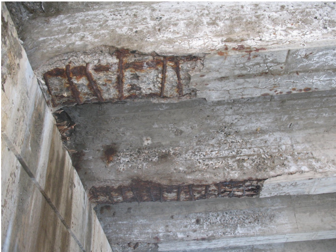
T-Beam deterioration.
