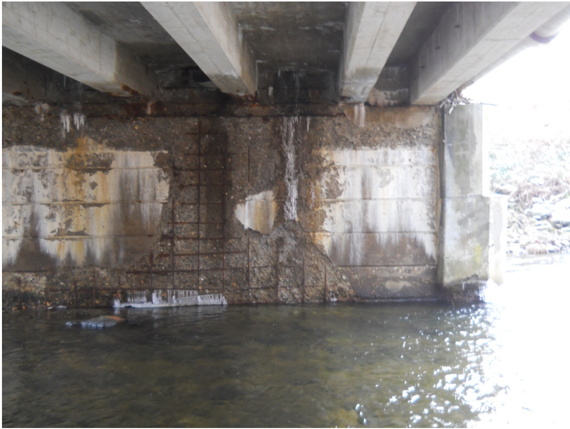
Substructure (Pier) deterioration
