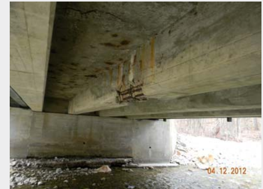
Exposed Rebar
