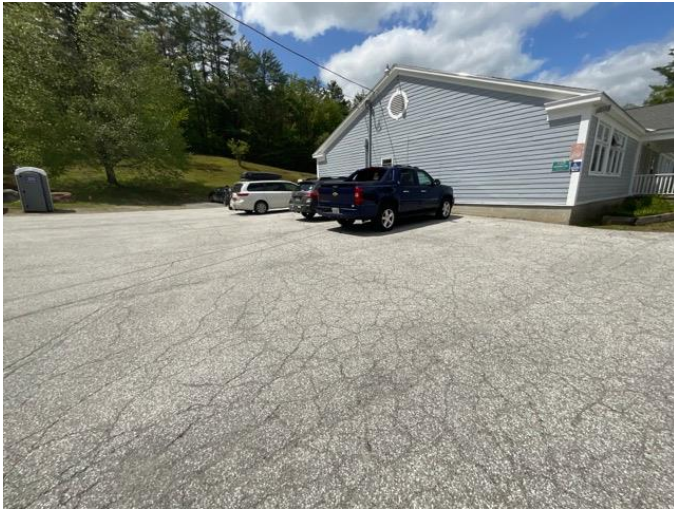
1 - OVERVIEW OF ACCESSIBLE PARKING AREA
