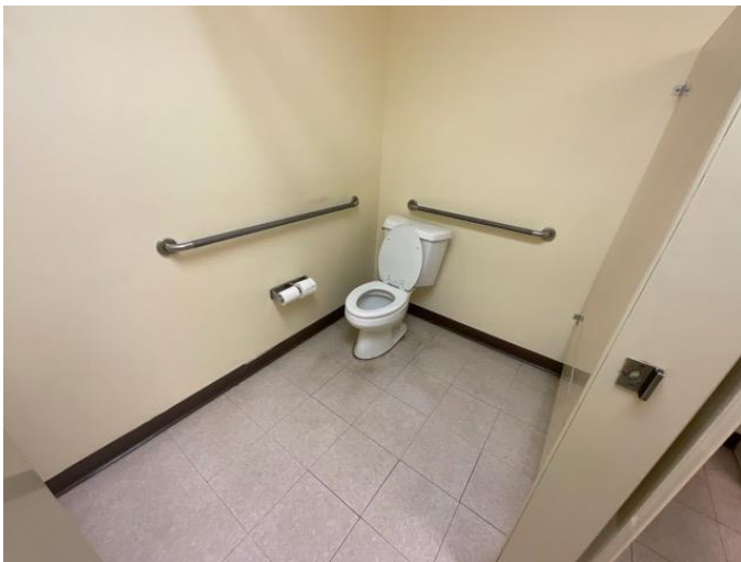
9 - TOILET STALL OVERVIEW
