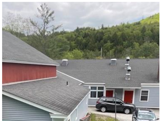
6 - MAIN ROOF OVERVIEW
