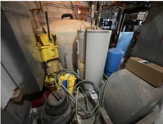
15 - ELECTRIC WATER HEATER
