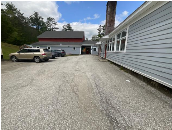
3 - OVERVIEW OF 2 ND PARKING AREA
