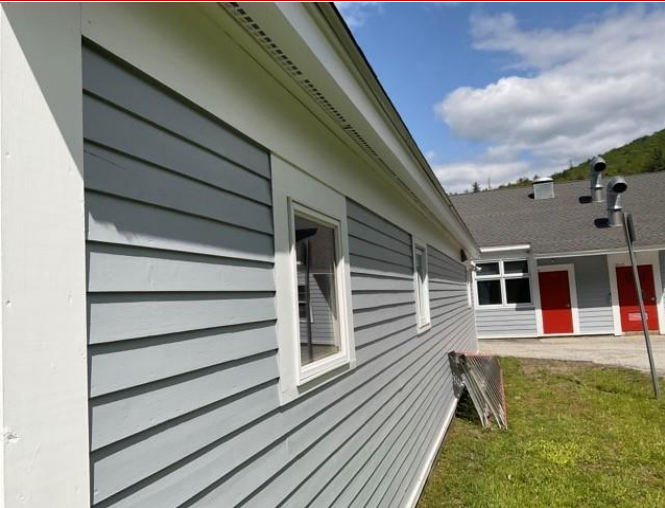
7 - PERIMETER ROOF AND DRAINAGE
