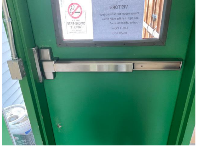
8 - HARDWARE, STAIR RAILS
