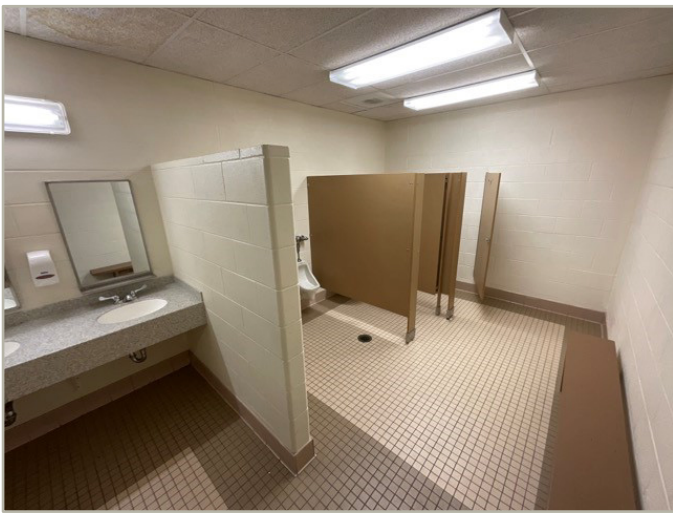
9 - TOILET STALL OVERVIEW
