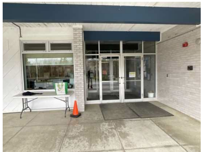
6 - MAIN BUILDING ENTRANCE
