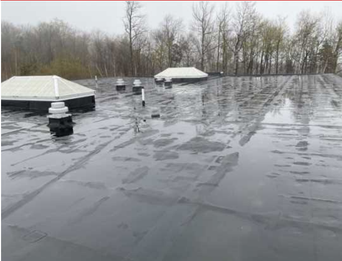
7 - PRIMARY EPDM ROOF OVERVIEW
