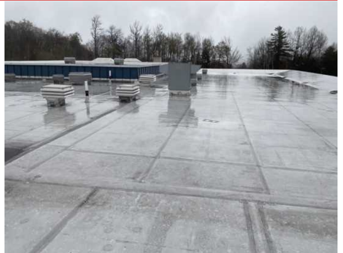
8 - SECONDARY TPO/PVC ROOF OVERVIEW
