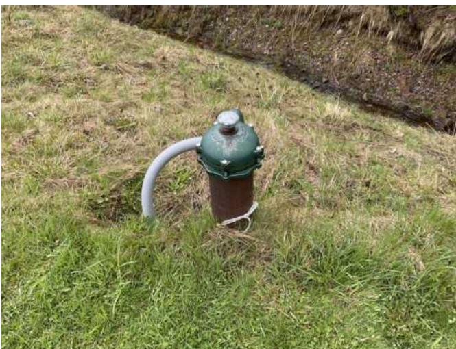
17 - PLUMBING SYSTEM WELL POINT
