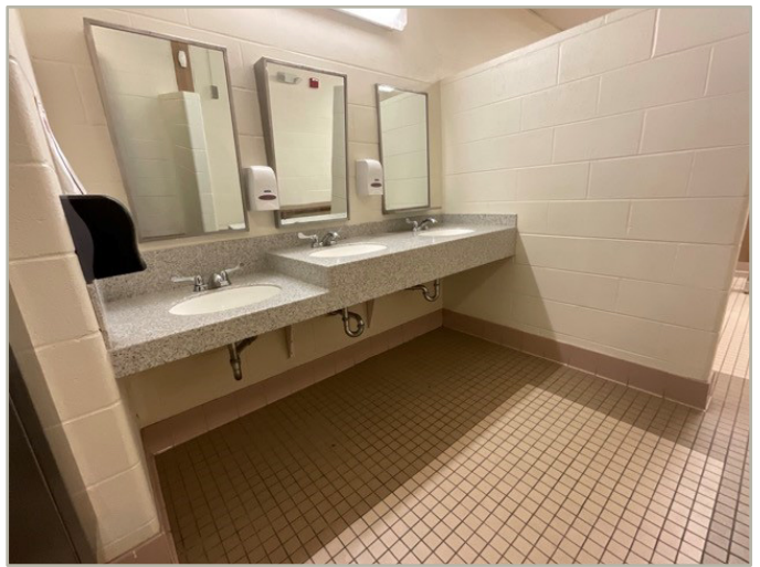
10 - SINK, FAUCET HANDLES
