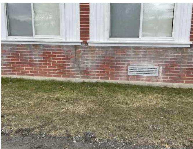
23 - EXTERIOR WALLS PHOTO
