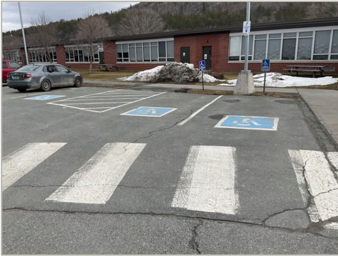
1 - OVERVIEW OF ACCESSIBLE PARKING AREA
