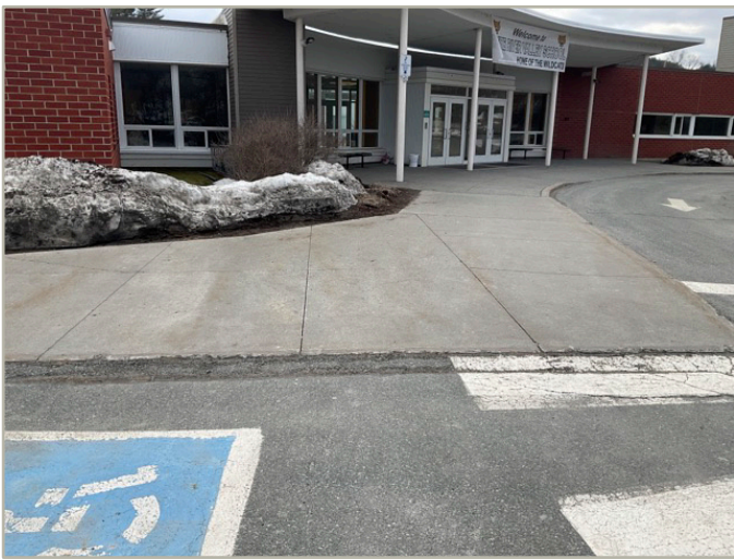
3 - EXT RAMP or PRIMARY PATH OF TRAVEL
