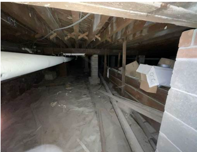
5 - SCHOOLS CRAWLSPACE FOUNDATION STRUCTURE
