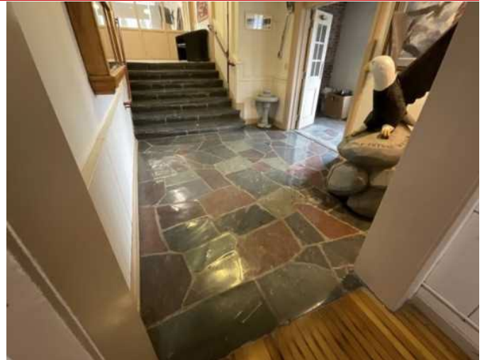
14 - INTERIOR SPACE ENTRANCE LOBBY
