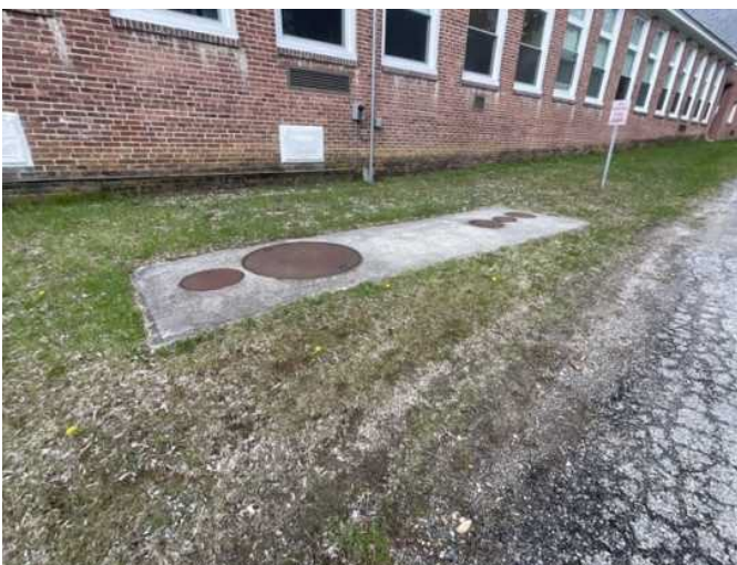
41 - FUEL OIL STORAGE TANK
