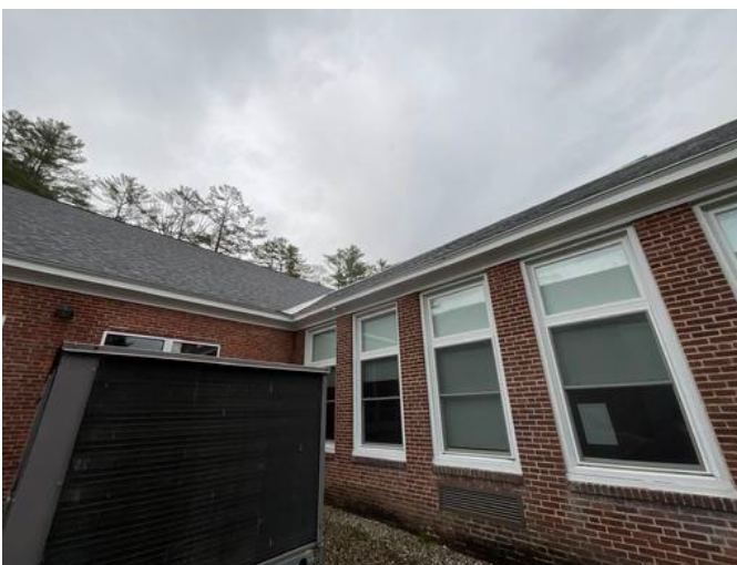
11 - ASPHALT SHINGLE ROOF TRANSITION
