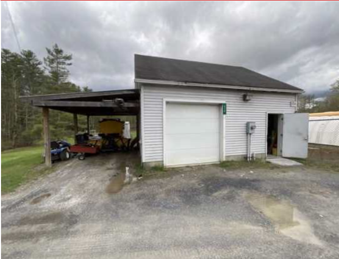
37 - SITE ANCILLARY STORAGE STRUCTURE
