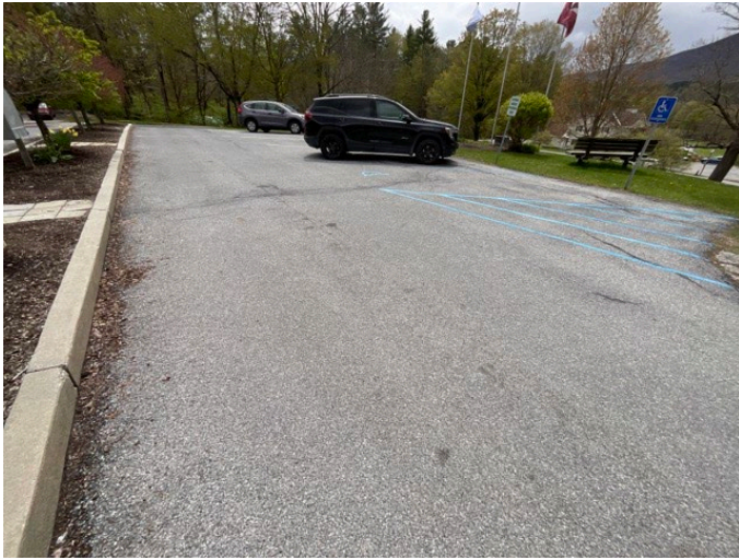
1 - OVERVIEW OF ACCESSIBLE PARKING AREA
