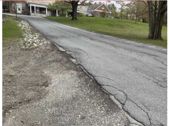
38 - SITE PAVED ROADWAY PHOTO
