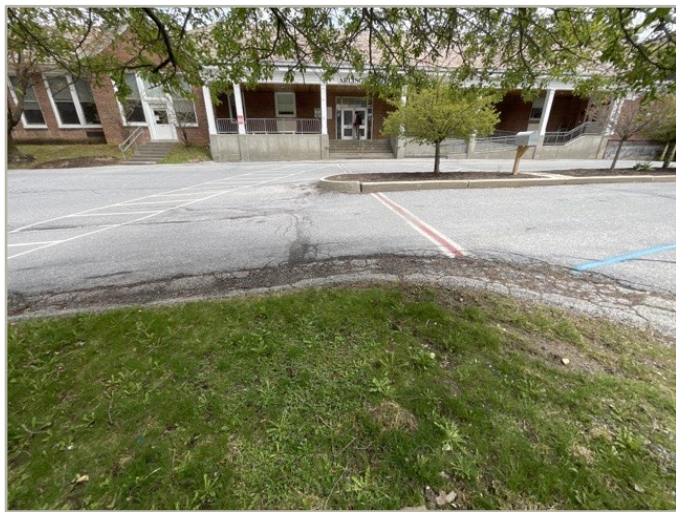
3 - EXT RAMP or PRIMARY PATH OF TRAVEL
