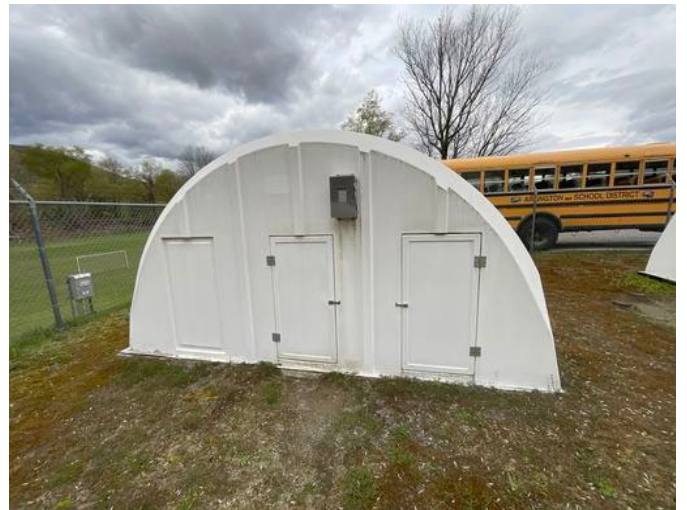
40 - WATER TREATMENT SEWAGE CONTAINER
