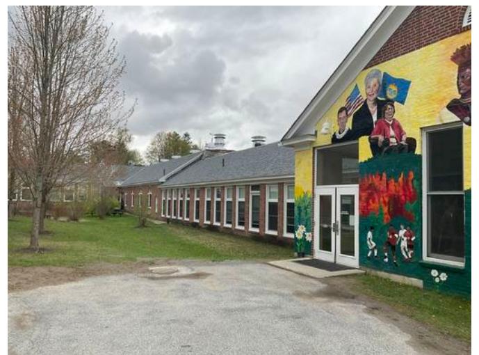
12 - ASPHALT SHINGLE ROOFING ON BUILDING
