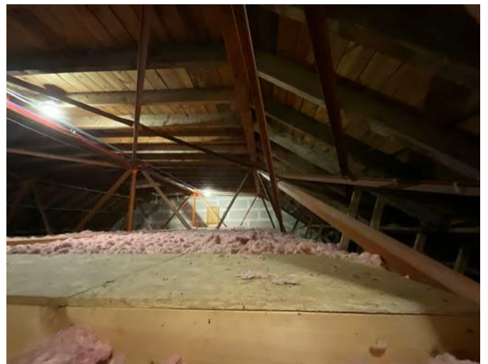
6 - SCHOOLS ATTIC AND ROOF STRUCTURE
