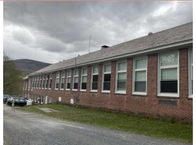
8 - SLATE ROOFING ON BUILDING
