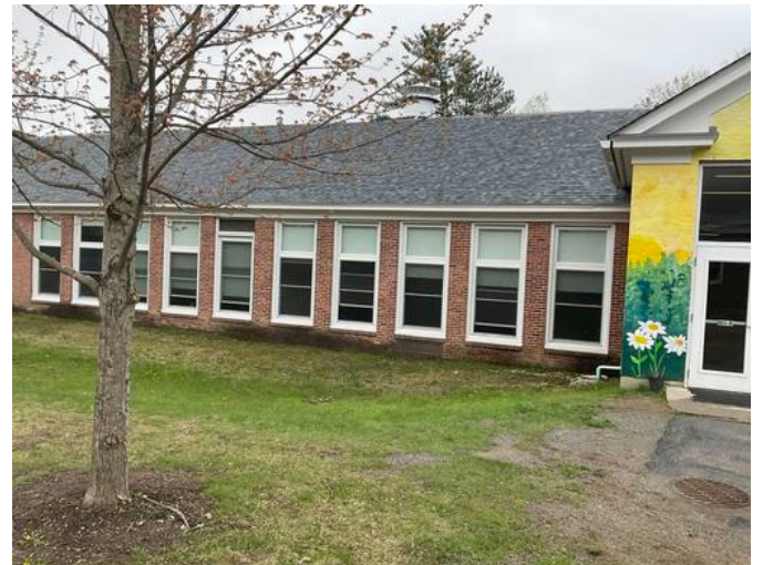
10 - ASPHALT SHINGLE ROOFING ON BUILDING
