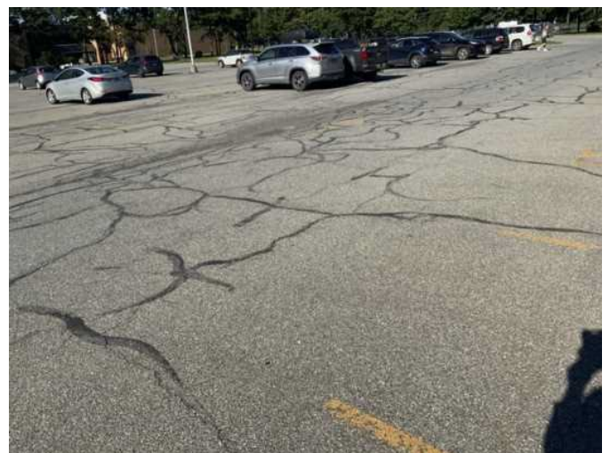
30 - PARKING LOT BETWEEN SCHOOLS
