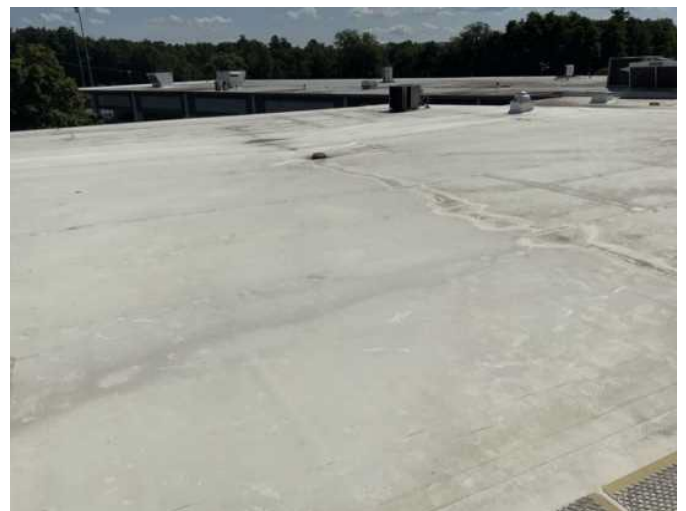
10 - TPO ROOF OVER CLASSROOM WING
