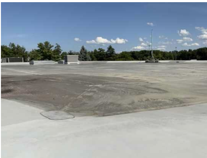
9 - FLAT ROOF TPO
