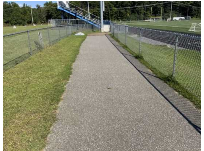
28 - ASPHALT WALKWAY AT STADIUM
