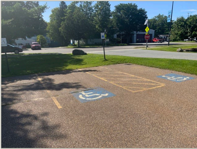
1 - OVERVIEW OF ACCESSIBLE PARKING AREA
