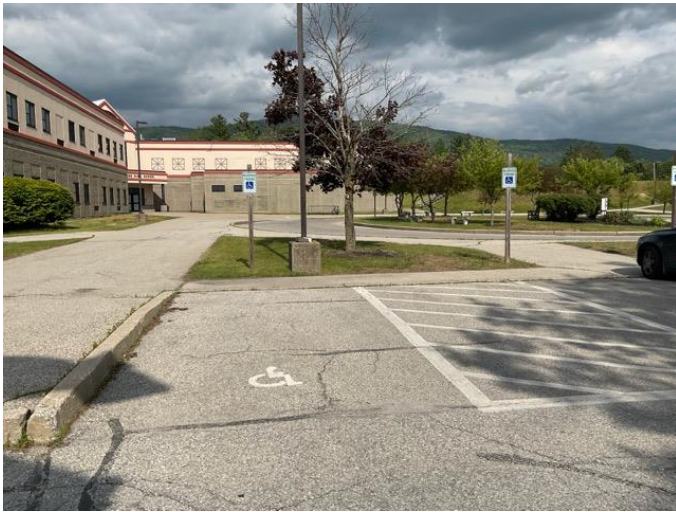
1 - OVERVIEW OF ACCESSIBLE PARKING AREA
