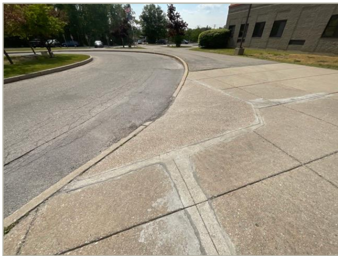
3 - EXT RAMP or PRIMARY PATH OF TRAVEL
