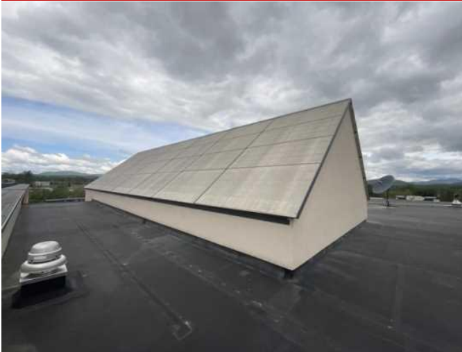
7 - GABLE STYLE KALWALL ROOF
