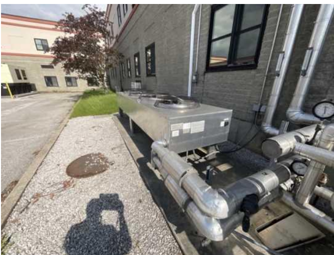
23 - COMPUTER ROOM AC UNIT
