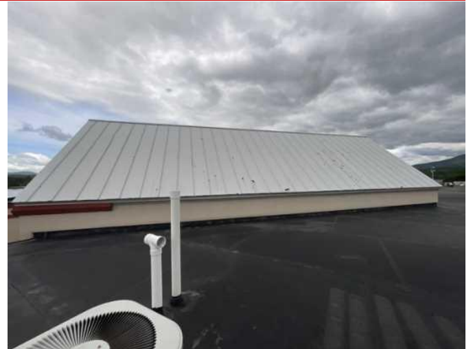
8 - GABLE STYLE METAL ROOF
