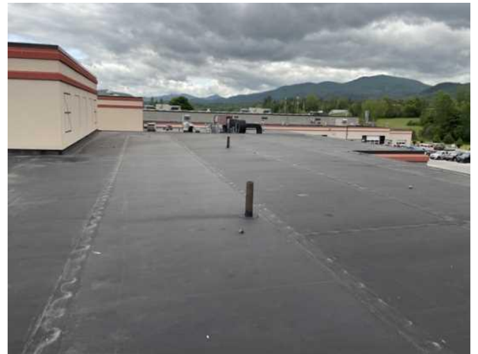
10 - FLAT ROOF OVERVIEW PHOTO
