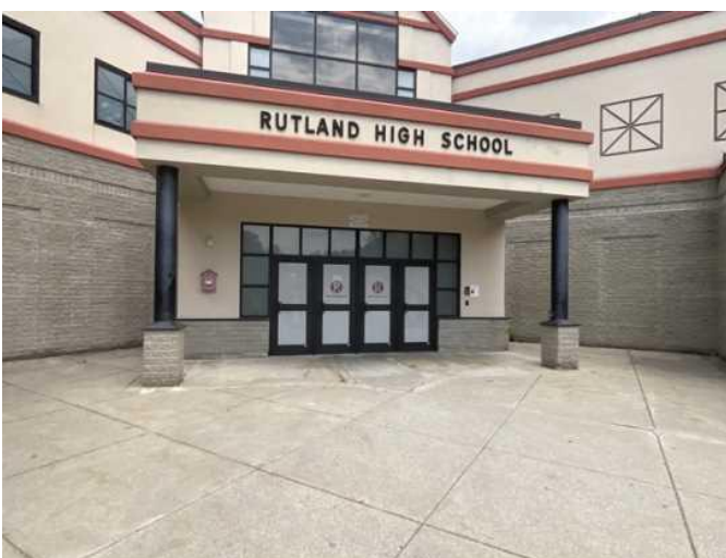
5 - EXTERIOR FAÇADE AND WINDOWS
