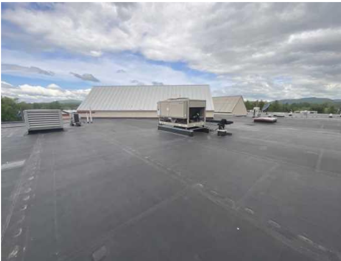
9 - FLAT ROOF OVERVIEW PHOTO
