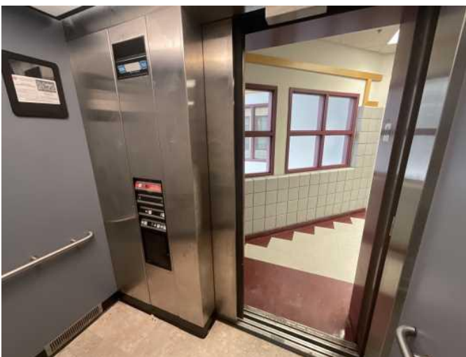
17 - CAB VIEW OF ELEVATOR
