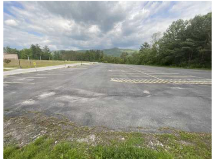
38 - ASPHALTS PAVED PARKING LOT
