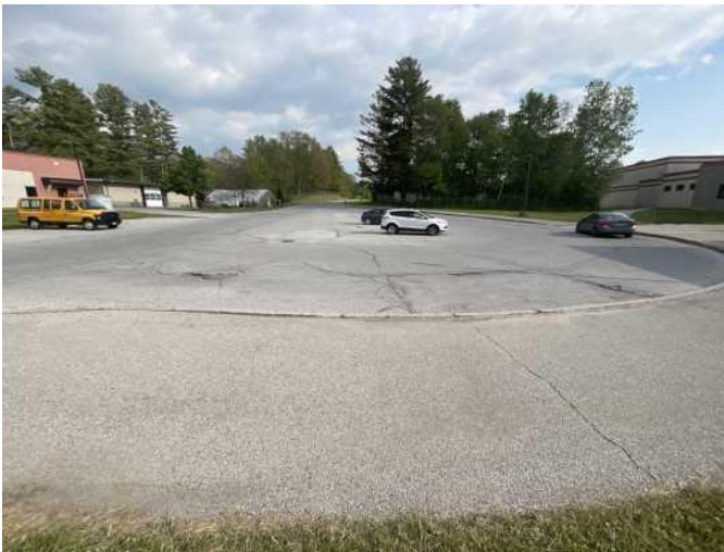
39 - ASPHALTS PAVED PARKING LOT
