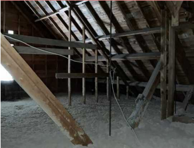
7 - STRUCTURAL LUMBER IN ATTIC
