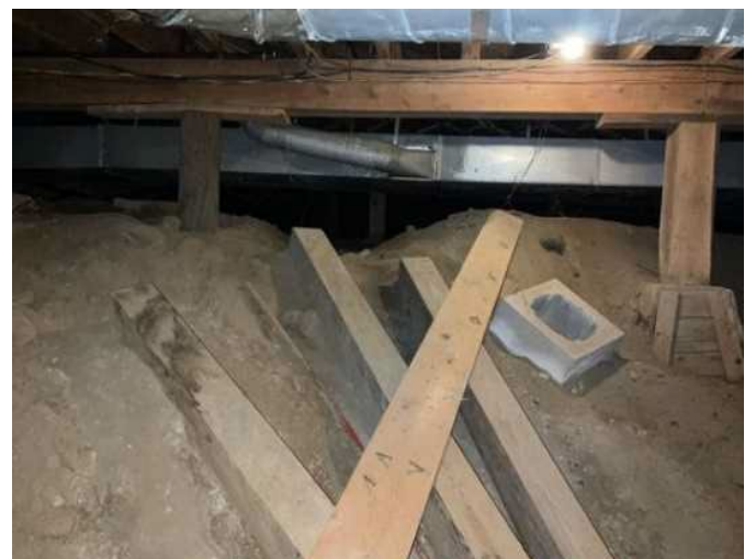
6 - CRAWLSPACE WITH STRUCTURAL LUMBER
