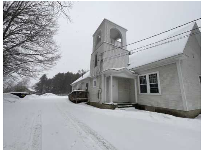
2 - LEFT ELEVATION OF SCHOOL
