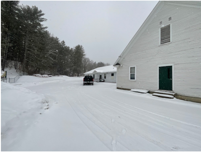
1 - OVERVIEW OF ACCESSIBLE PARKING AREA
