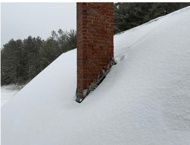
11 - ROOF WITH BRICK CHIMNEY
