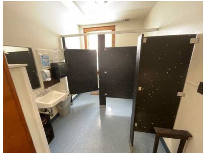
22 - TOILET PARTITIONS IN RESTROOM
