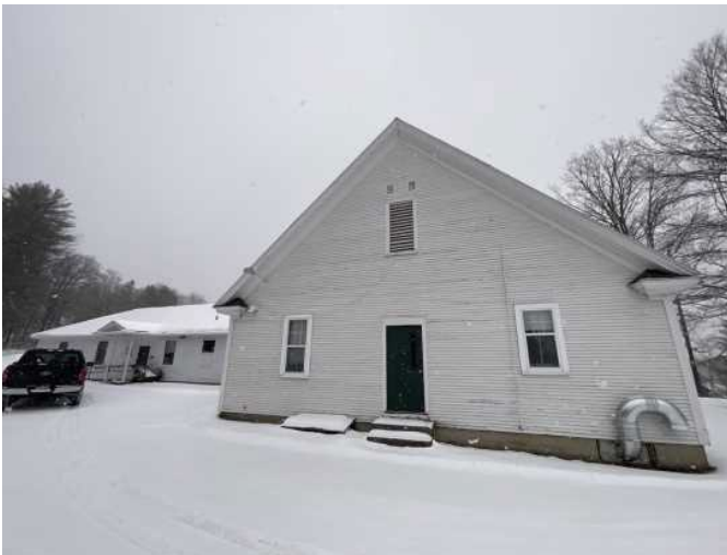
3 - REAR ELEVATION OF SCHOOL
