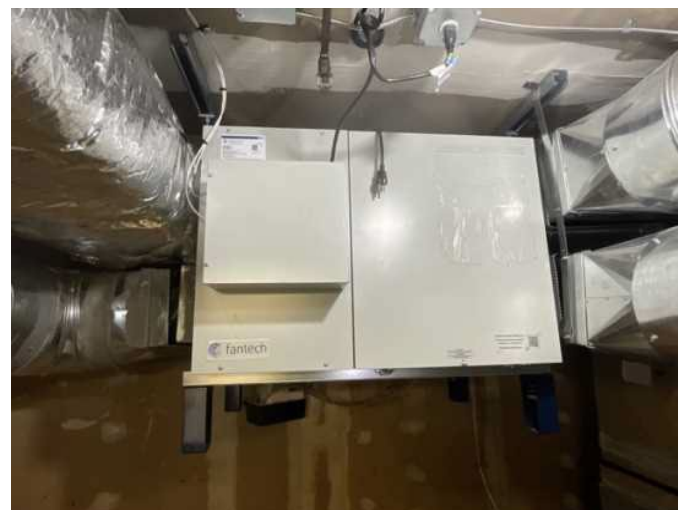
18 - HEAT RECOVERY VENTILATOR UNIT
