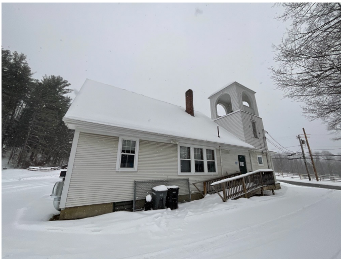
3 - EXT RAMP or PRIMARY PATH OF TRAVEL
