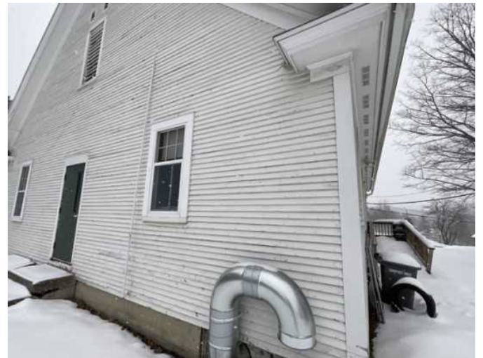
10 - EXTERIOR WALLS WOOD SIDING
