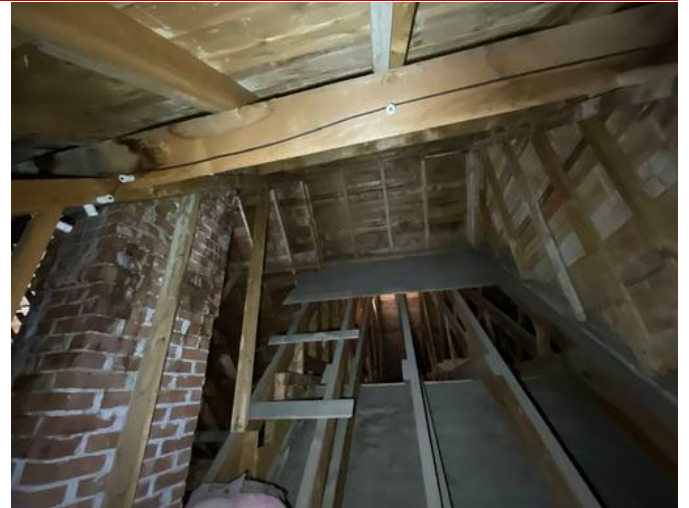
8 - STRUCTURAL LUMBER OF ROOF
