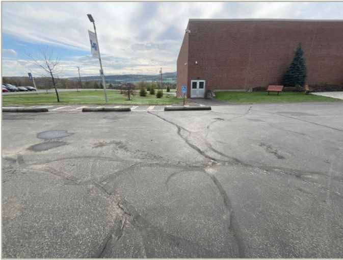
1 - OVERVIEW OF ACCESSIBLE PARKING AREA
