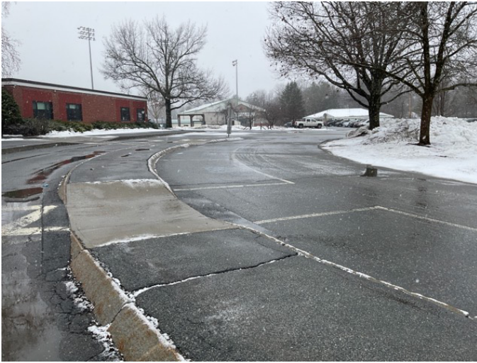
1 - OVERVIEW OF ACCESSIBLE PARKING AREA
