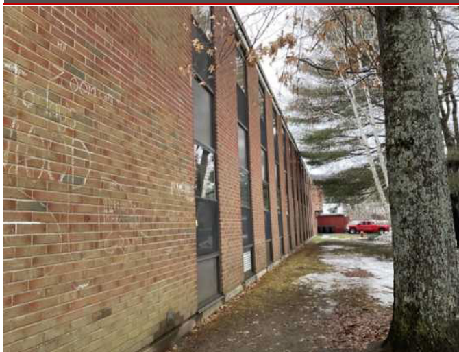
7 - BRICK VENEER, METAL PANELS AND ALUMINUM
