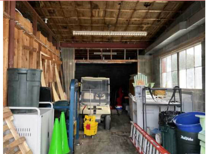
14 - BUS BARN INTERIOR
