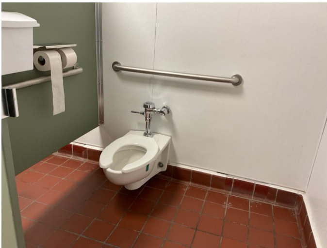
9 - TOILET STALL OVERVIEW
