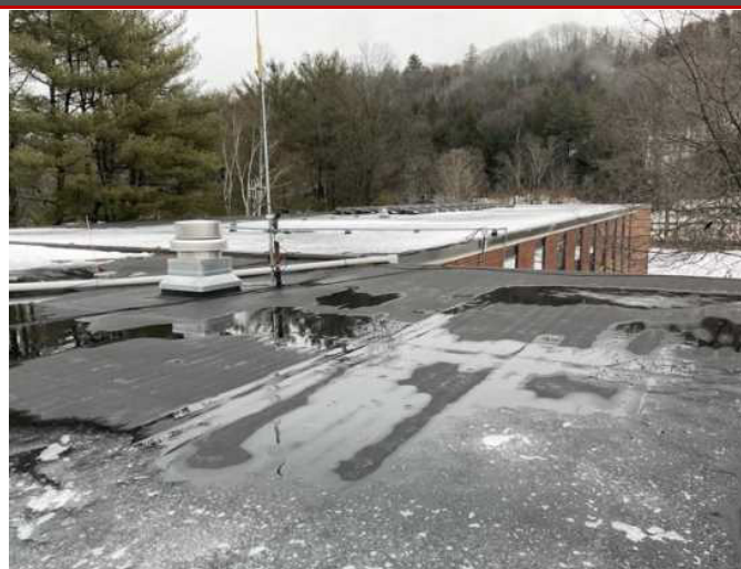
8 - PRIMARY ROOF OVERVIEW
