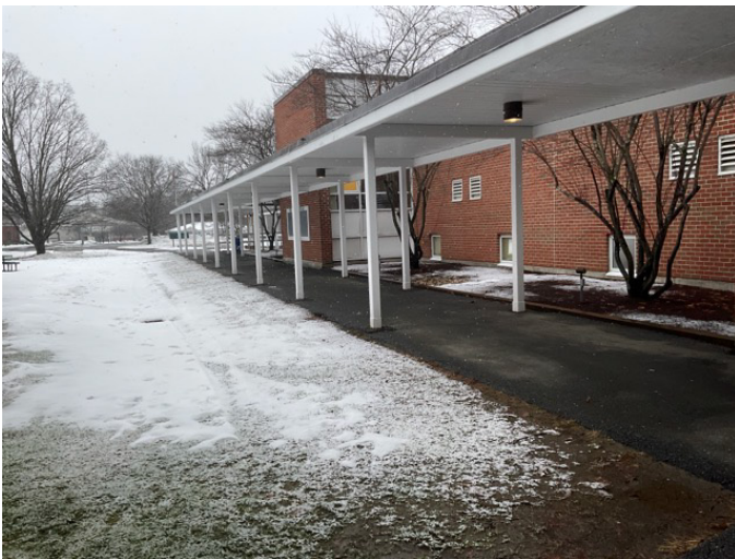
3 - EXT RAMP or PRIMARY PATH OF TRAVEL
