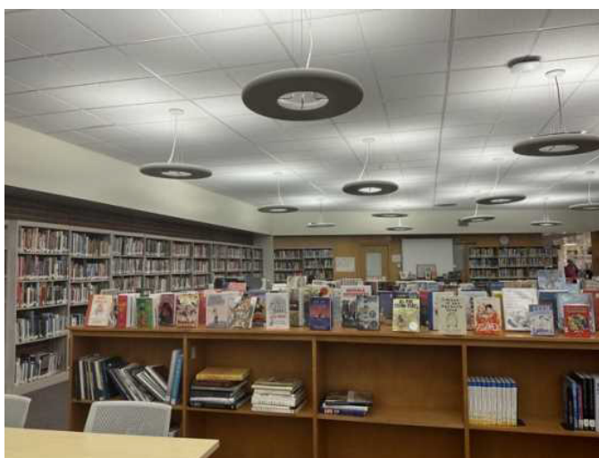
11 - UPGRADED CEILING AND LIGHTING AT LIBRARY
