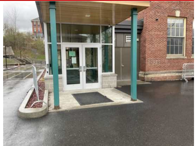
8 - RECENTLY ADDED ACCESSIBLE ENTRANCE
