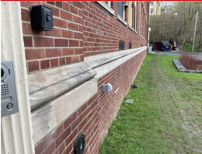
7 - BRICK MORTAR JOINTS OVERVIEW
