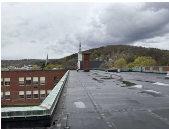
9 - FLAT EPDM ROOF OVERVIEW
