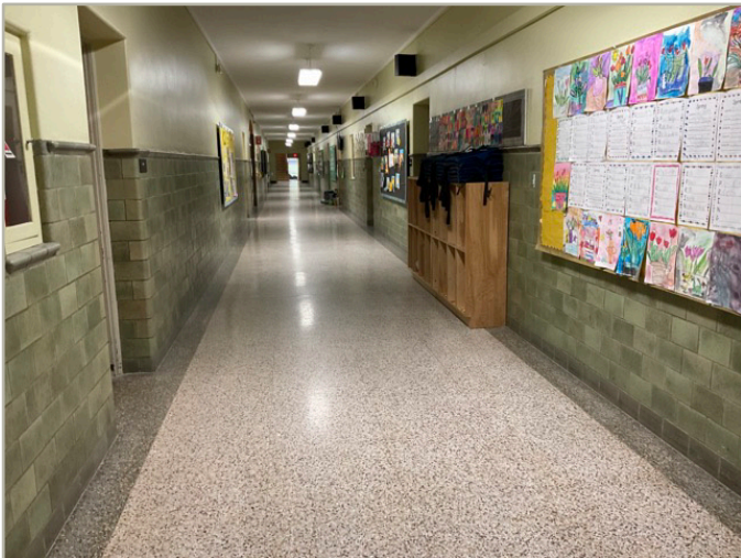
5 - ACCESSIBLE INTERIOR PATH (RAMP/LIFT)
