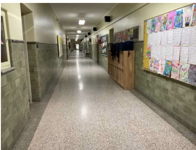
11 - OVERVIEW OF HALLWAY SURFACES
