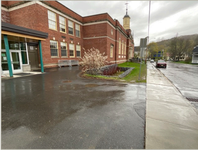
1 - EXT RAMP or PRIMARY PATH OF TRAVEL
