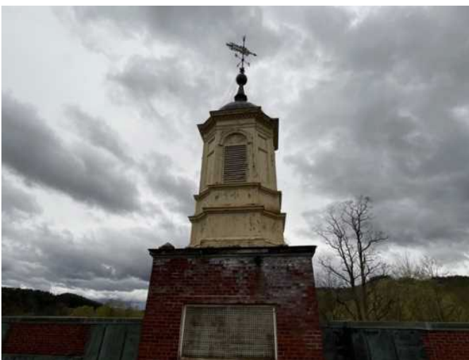
5 - ENTRANCE STEEPLE FROM ROOF
