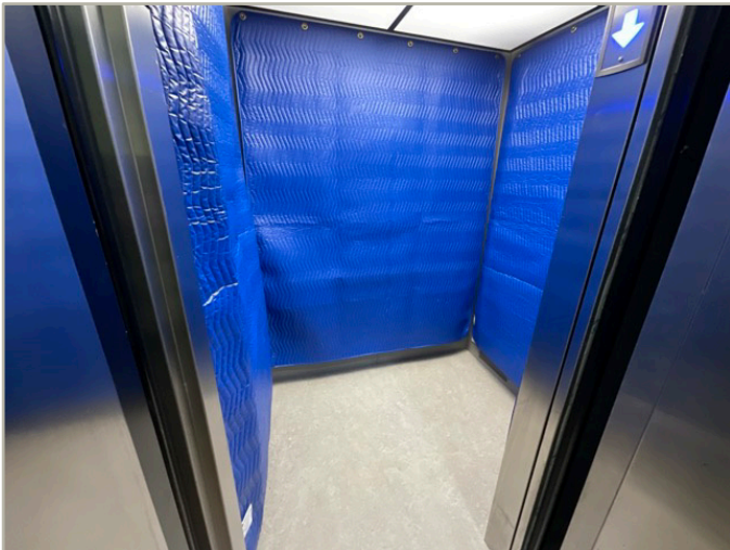
11 - LOBBY VIEW OF CABS, WITH DOORS OPEN
