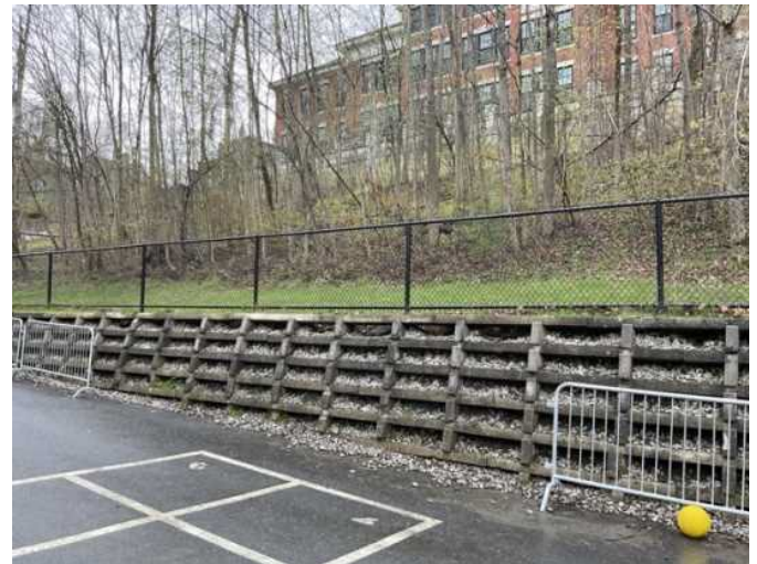
28 - DRAINABLE CONCRETE RETAINING WALL
