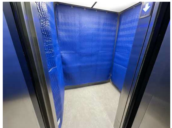
10 - ELEVATOR CAB INTERIOR OVERVIEW
