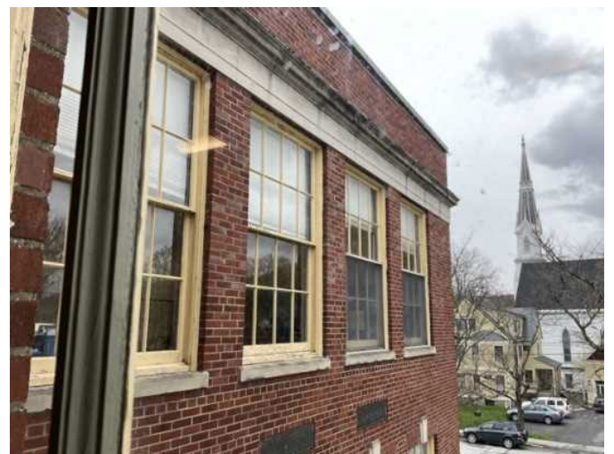
6 - OVERVIEW OF EXTERIOR WINDOWS
