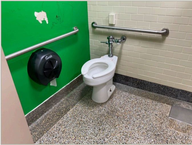
7 - TOILET STALL OVERVIEW
