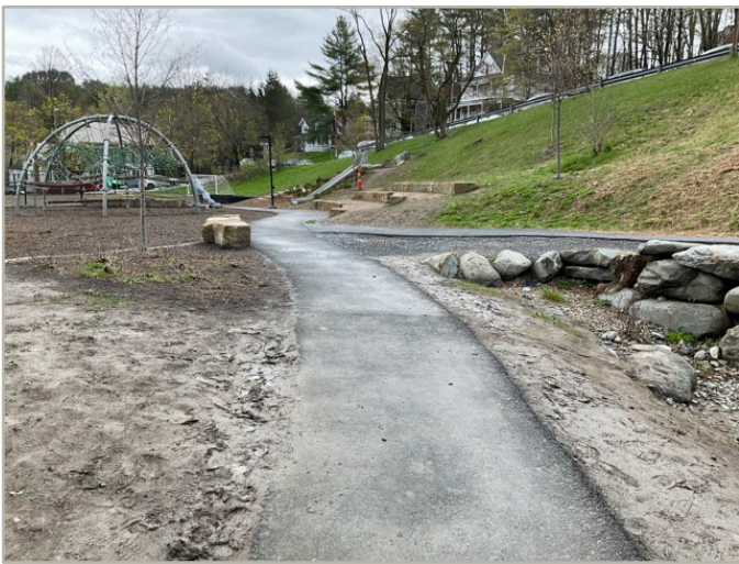
9 - ACCESSIBLE ROUTE TO PLAYGROUND
