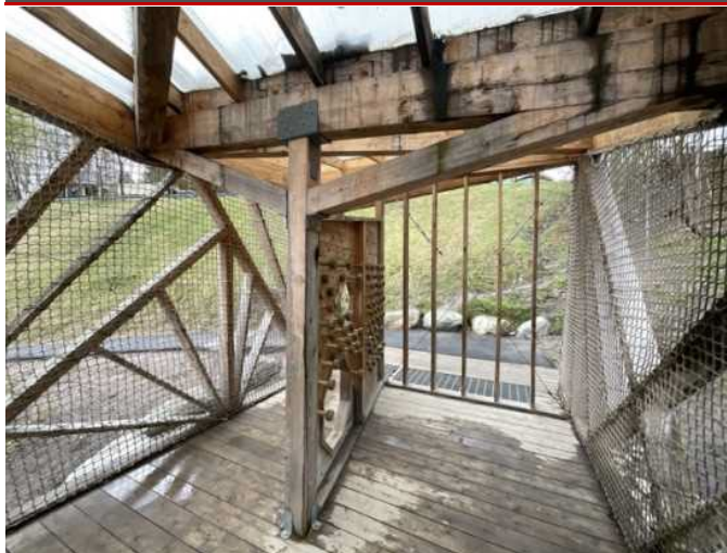
31 - INTERIOR OF PLAY STRUCTURE
