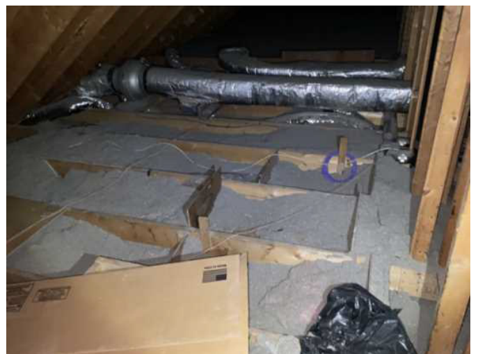
6 - ATTIC FRAMING AND SPACE
