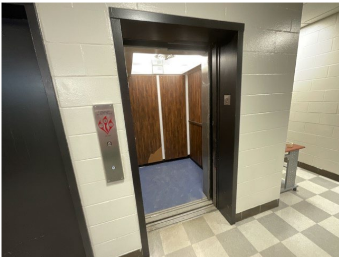
13 - LOBBY VIEW OF CABS, WITH DOORS OPEN
