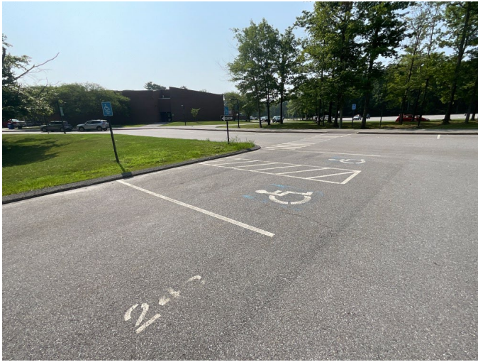
1 - OVERVIEW OF ACCESSIBLE PARKING AREA
