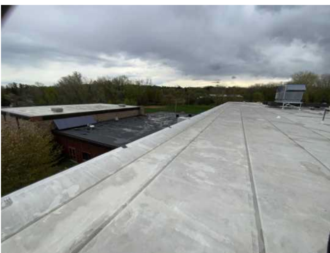
5 - PHOTO OF AN OVERALL ROOFING
