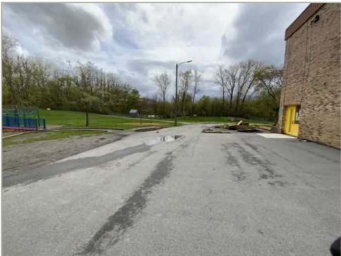
11 - ACCESSIBLE ROUTE TO PLAYGROUND
