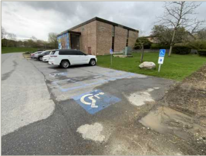
1 - OVERVIEW OF ACCESSIBLE PARKING AREA
