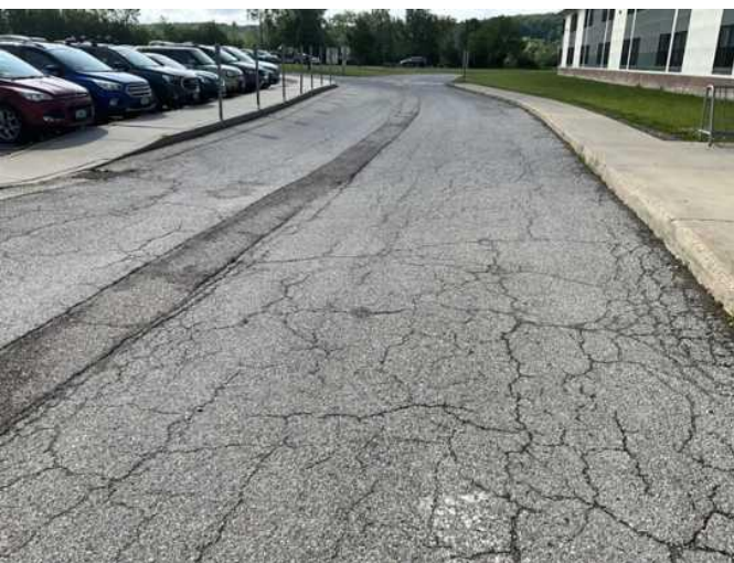
59 - PARKING LOT AND ROAD WAY PAVEMENT
