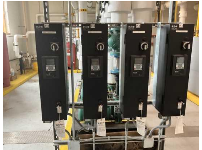
52 - MOTOR VARIABLE FREQUENCY DRIVES
