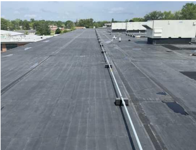
9 - EPDM ROOFING A WING AND D WING
