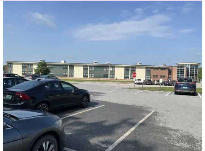
2 - LEFT ELEVATION OF BUILDING
