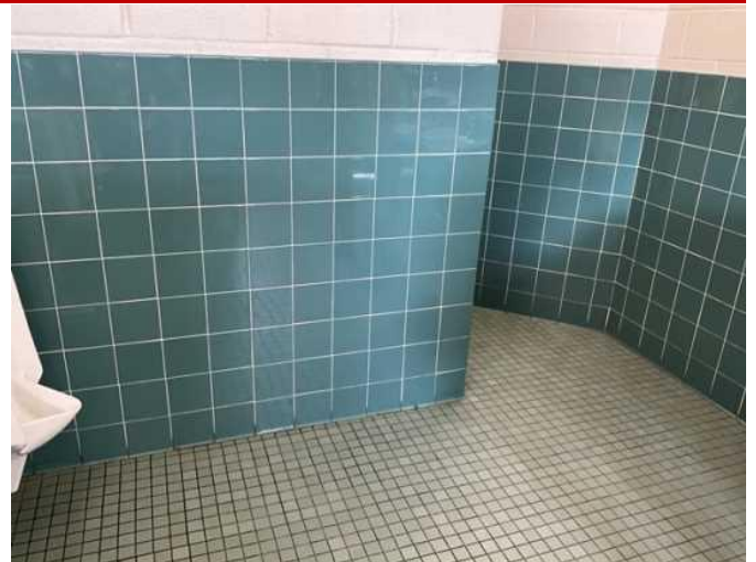
20 - RESTROOM WALLS CERAMIC TILE
