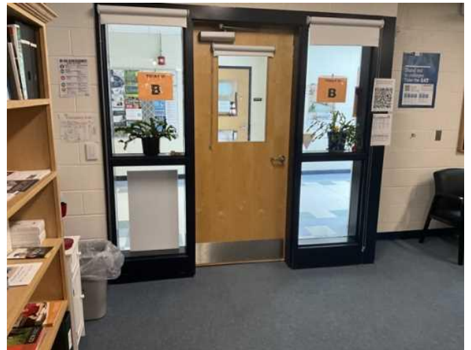
16 - CLASSROOM/OFFICES INTERIOR DOOR
