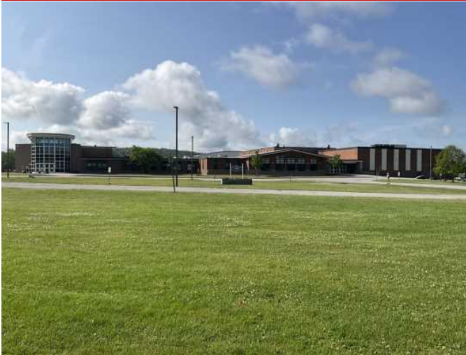
1 - FRONT ELEVATION OF BUILDING
