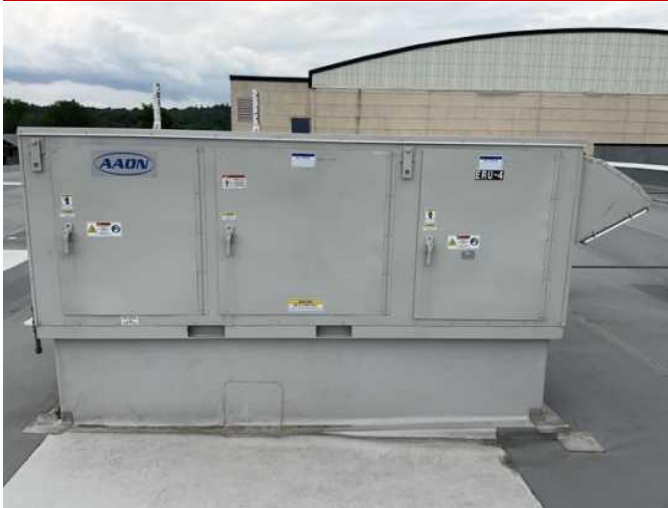
43 - ENERGY RECOVERY AIR VENTILATOR
