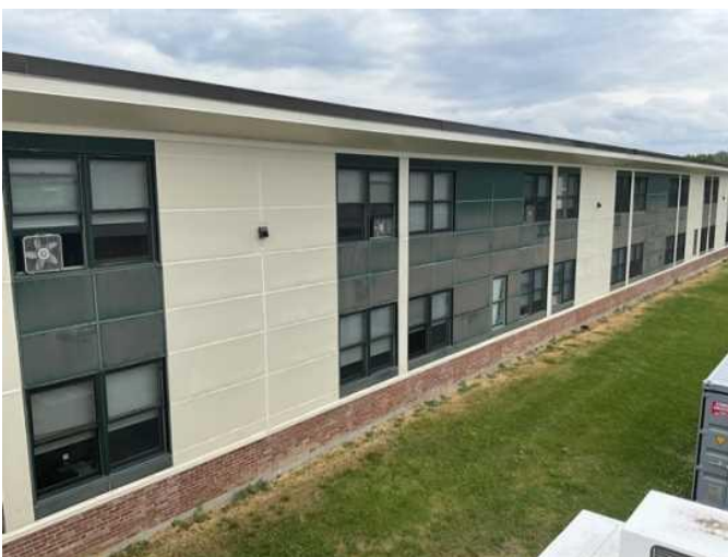
11 - EXTERIOR WALLS C/D WING
