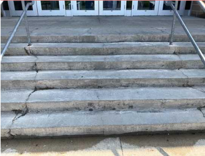
7 - STAIRS TO GYMNASIUM ENTRANCE
