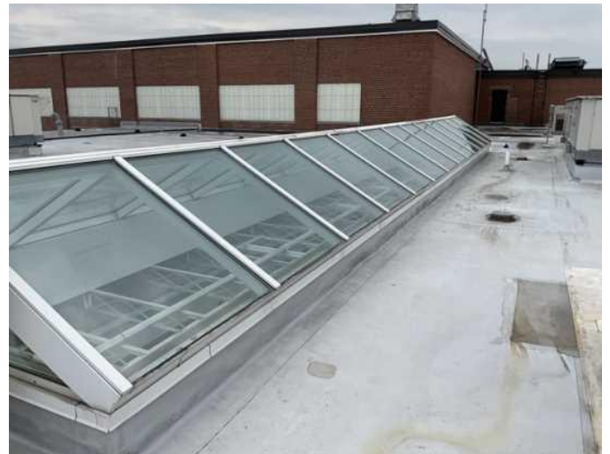
10 - CAFETERIA ROOF SKYLIGHT OVERVIEW
