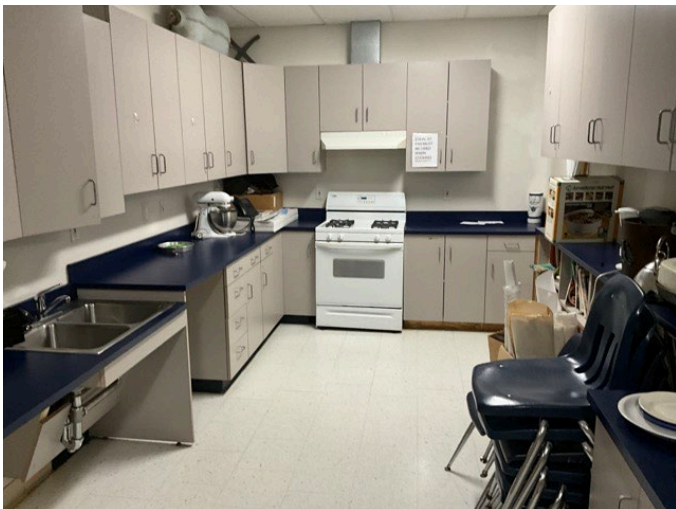
15 - KITCHEN CABINETS/SINK CLEARANCE
