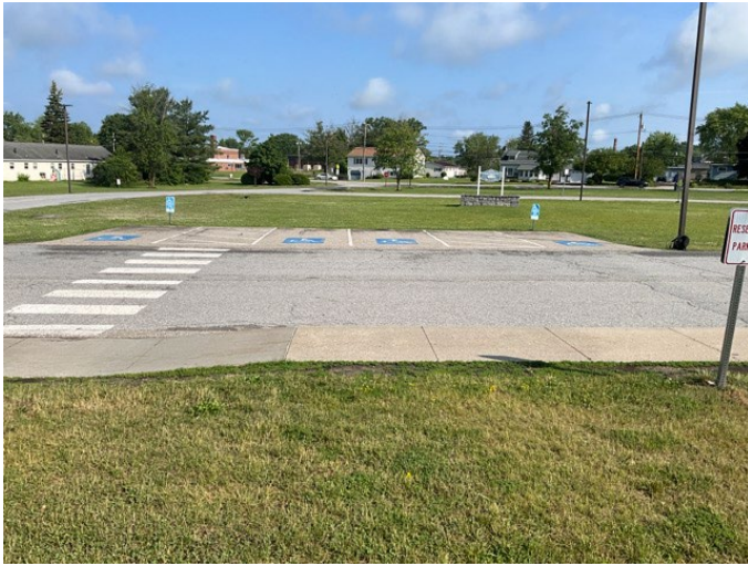
1 - OVERVIEW OF ACCESSIBLE PARKING AREA
