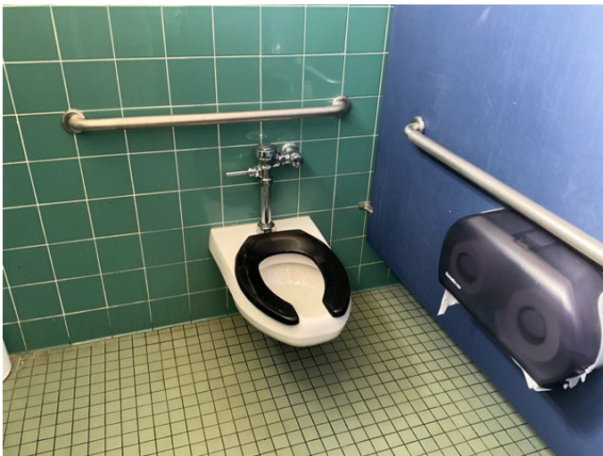
9 - TOILET STALL OVERVIEW
