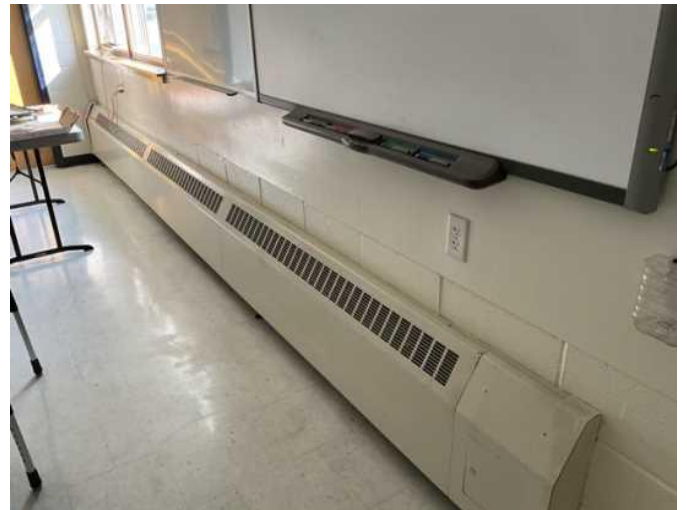
40 - HYDRONIC BASE BOARD HEATER
