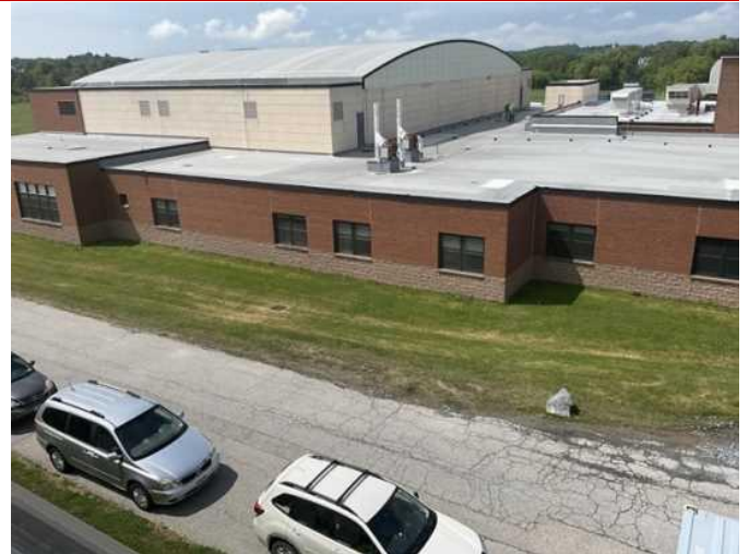
8 - EXTERIOR WALLS AND TPO ROOFING B AND C
