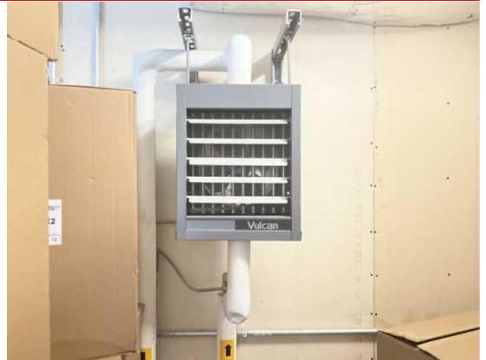
44 - HYDRONIC COIL UNIT HEATER
