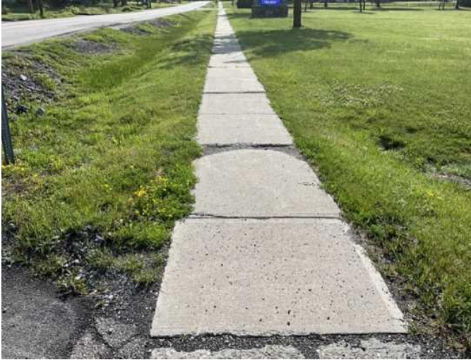
61 - SITE CONCRETE SIDEWALK/ WALKWAY
