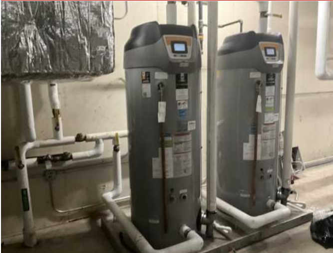
25 - HIGH EFFICIENCY WATER HEATER
