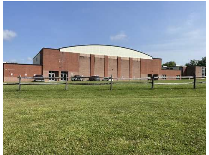
4 - REAR ELEVATION OF BUILDING
