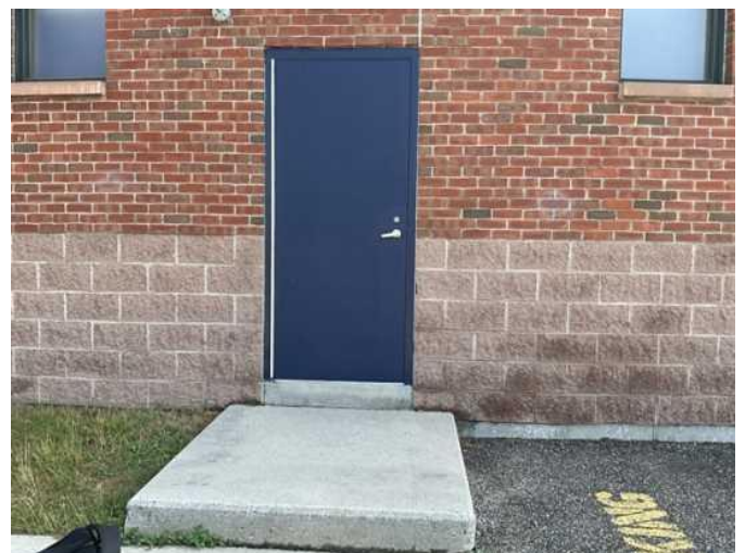
12 - BUILDING EXTERIOR STEEL DOOR
