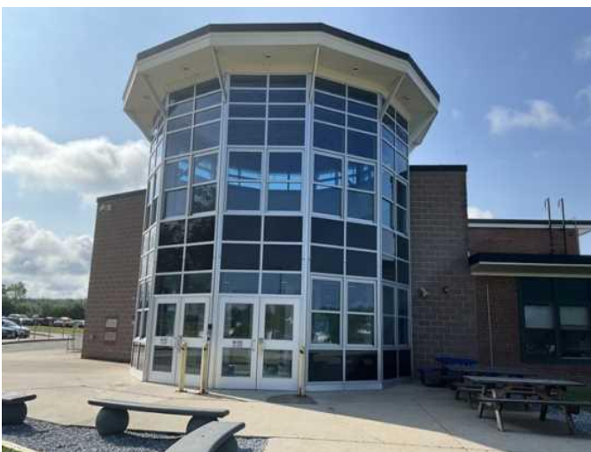
5 - MAIN ENTRANCE DOORS AND GLAZING
