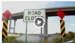
Building a Bridge to Reduce Risk Watch video >
