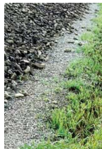
Verges built according to accepted standards, and in combination with a grass-covered and regularly mown transition band can be an ideal vegetation barrier against weed incursions.
