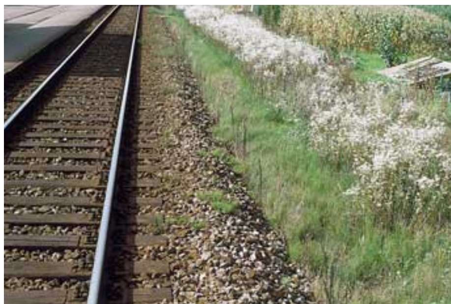
The best approach is generally a combination of methods, to ensure that gaps left in the vegetation are not taken up by other unwanted plant species. The example in the picture shows that a one-sided treatment with herbicides extremely favours the propagation of horsetail!
