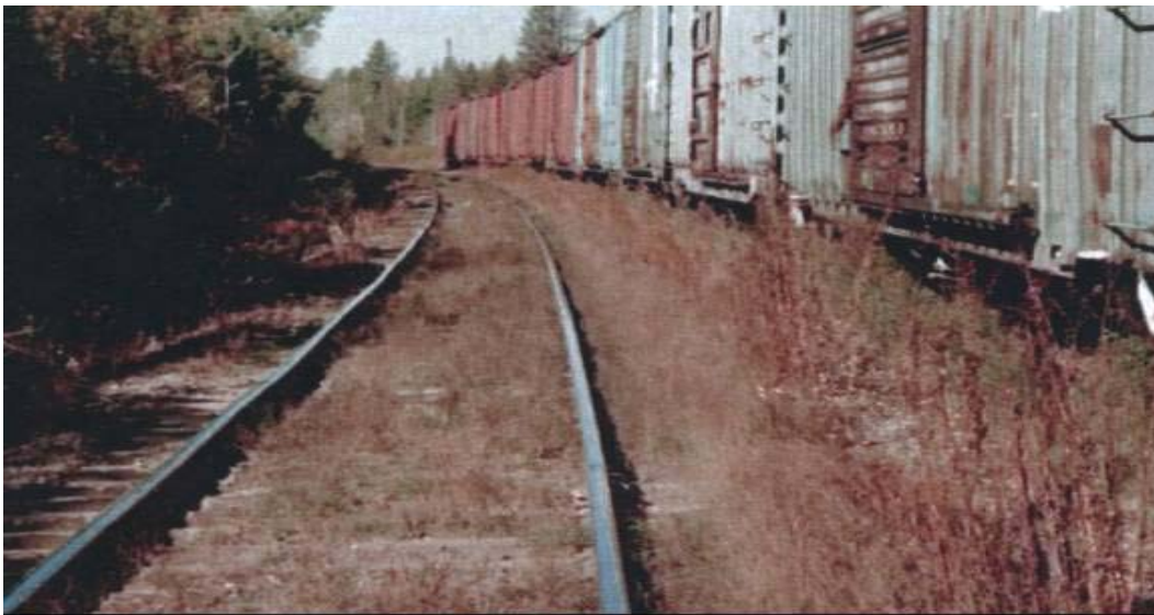
Figure 10 Typical “intensive treatment” track condition.
