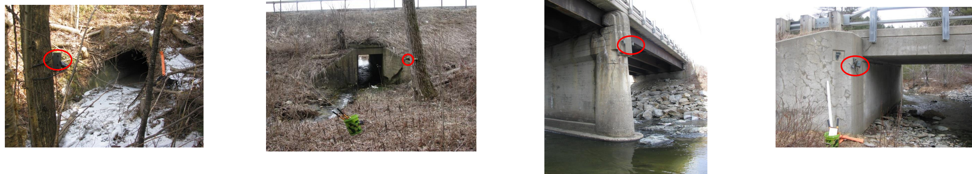
Figure 1. Examples of game camera positioning at monitored transportation structures.
