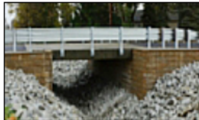
Geosynthetic Reinforced Soil-Integrated Bridge System
