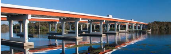
Accelerated Bridge Construction (ABC)
