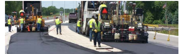
Warm Mix Asphalt
