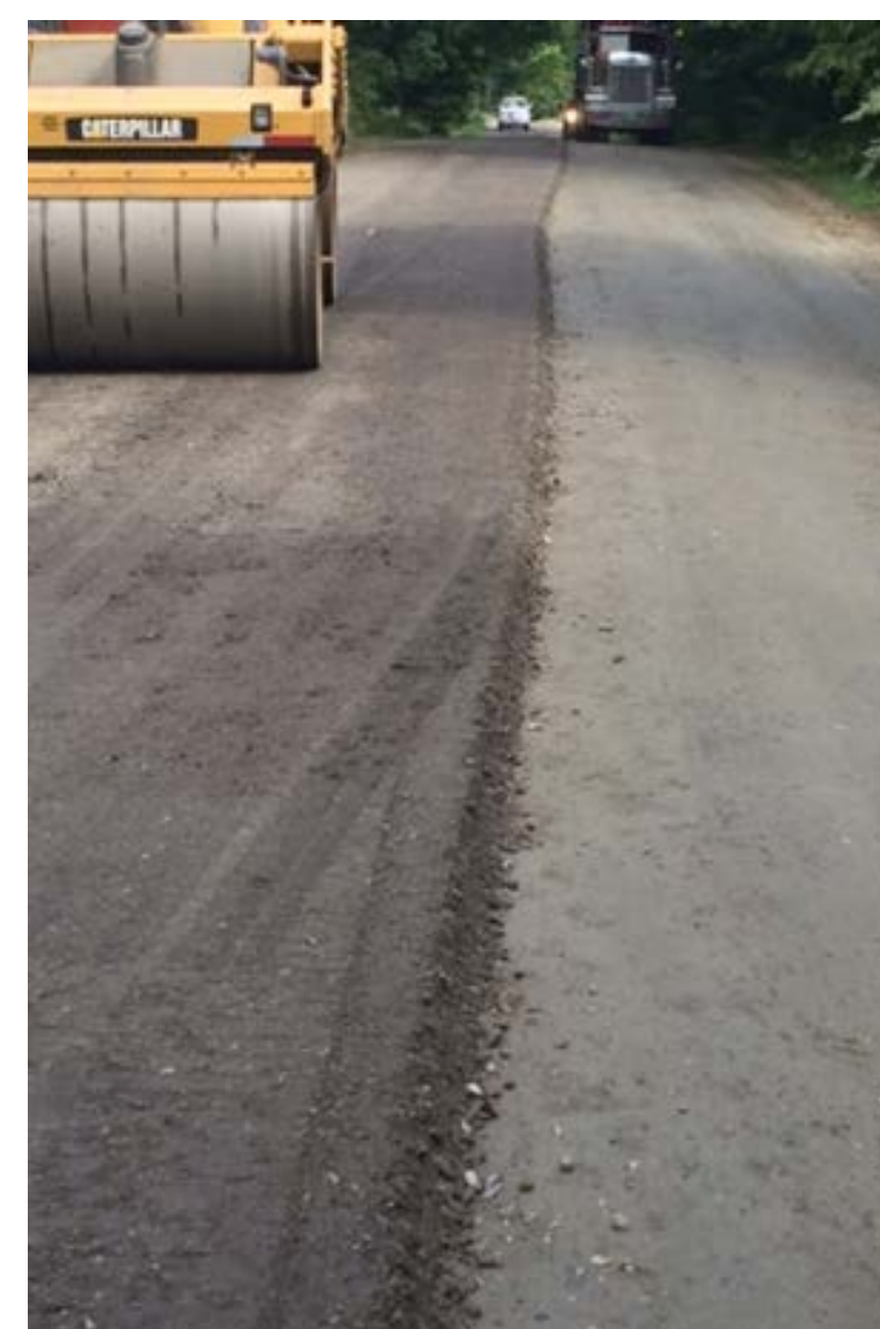
Gravel / RAS Surface Mix on VT 65 in Brookfield
