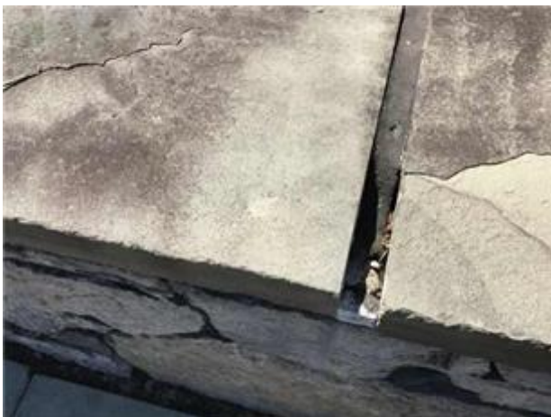
Failed sealant
