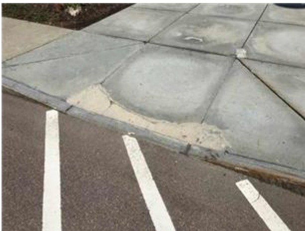
Deteriorated pavers
