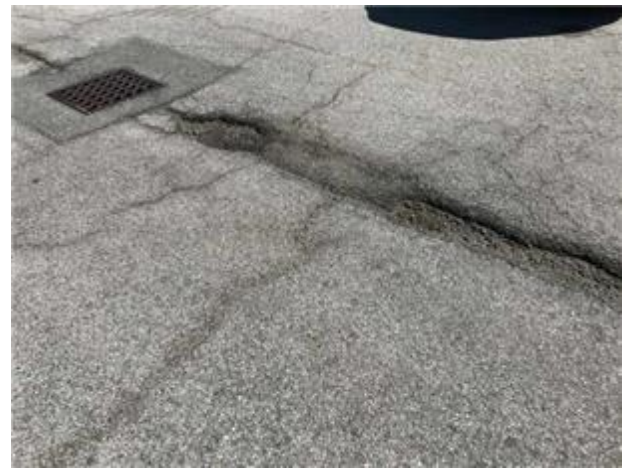
Asphalt wear
