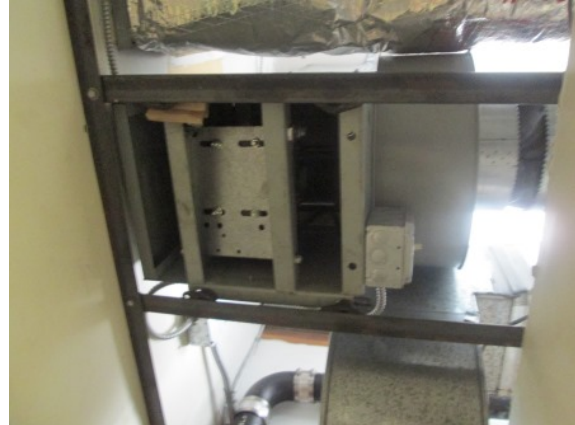
Photo #26: Typical exhaust fan
