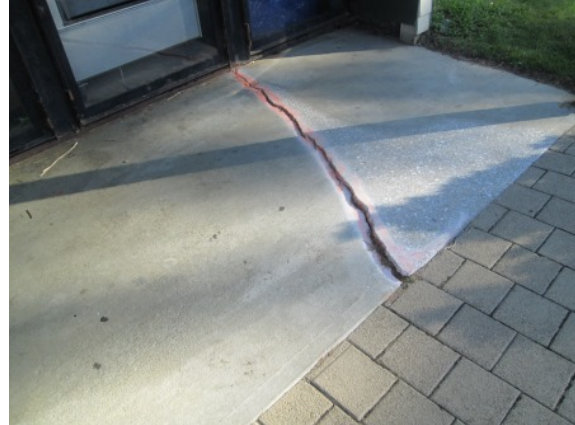
Photo #10: Northbound vending area foundation with crack and settlement
