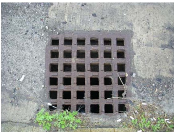
Outfall 252A: 24" CMP
