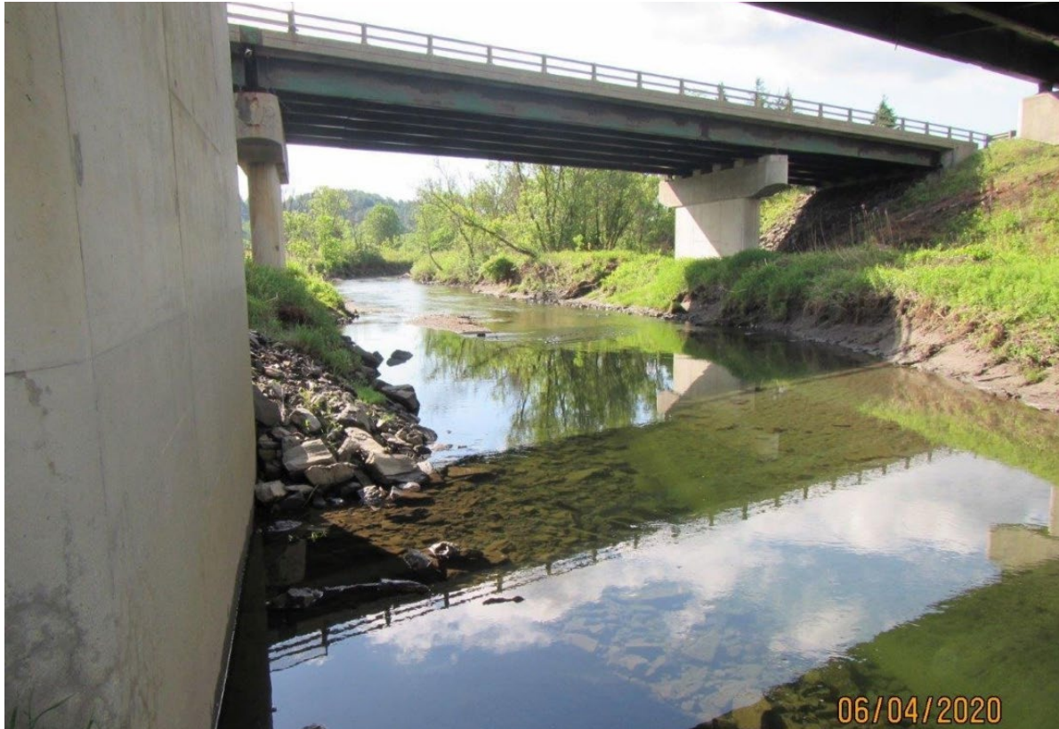
Photograph 28: Bridge 0096N. Map ID 24. Photograph taken by VTrans June 4, 2020.
