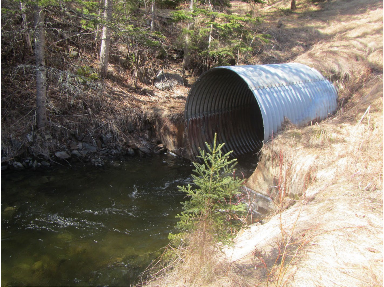
Photograph 21: Culvert 96-3N Map ID 18
