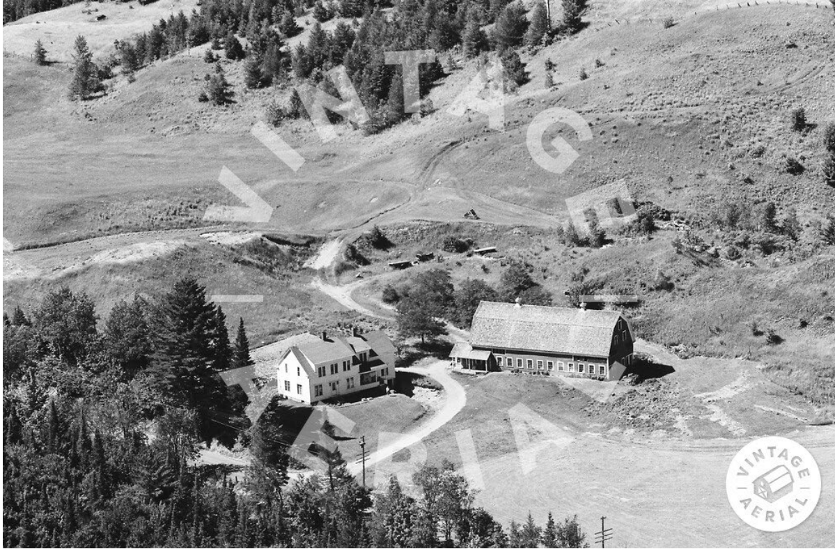
Figure: 374 VT Route 122. The barn to the right of the house is no longer extant but the house remains today. Vintage Aerial Photograph 4-QCA-7.
