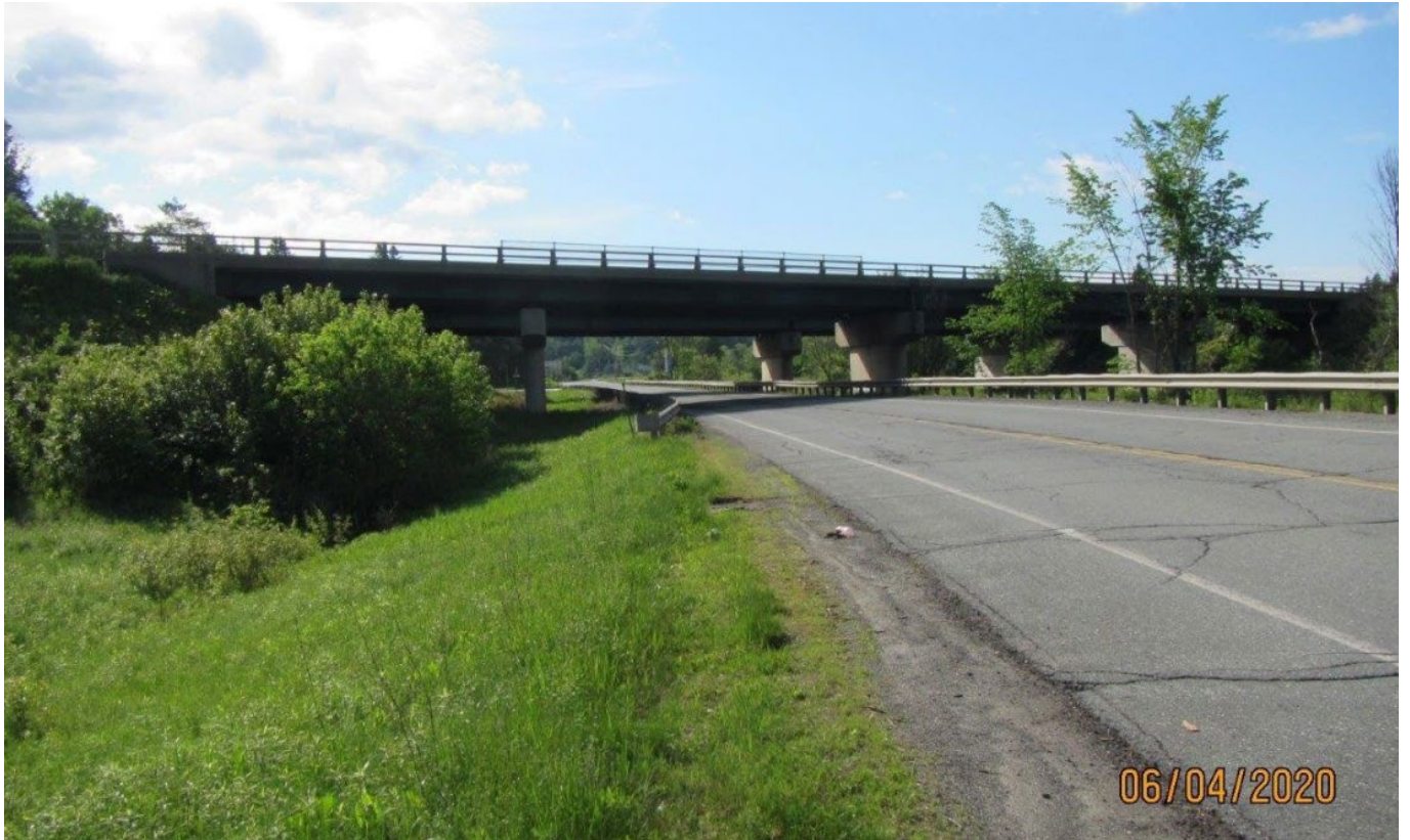
Photograph 29: Bridge 0096S. Map ID 25. Photograph taken by VTrans June 4, 2020.
