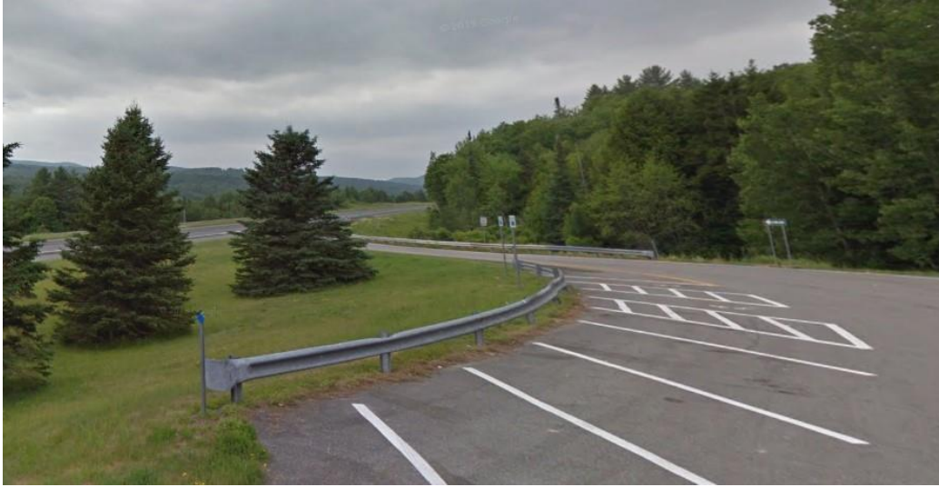
Figure 13. South view of the rest stop at the north APE segment showing one location within the proposed VTrans Lyndon IM 091-3(53) Project, Lyndon, Caledonia County, Vermont.
