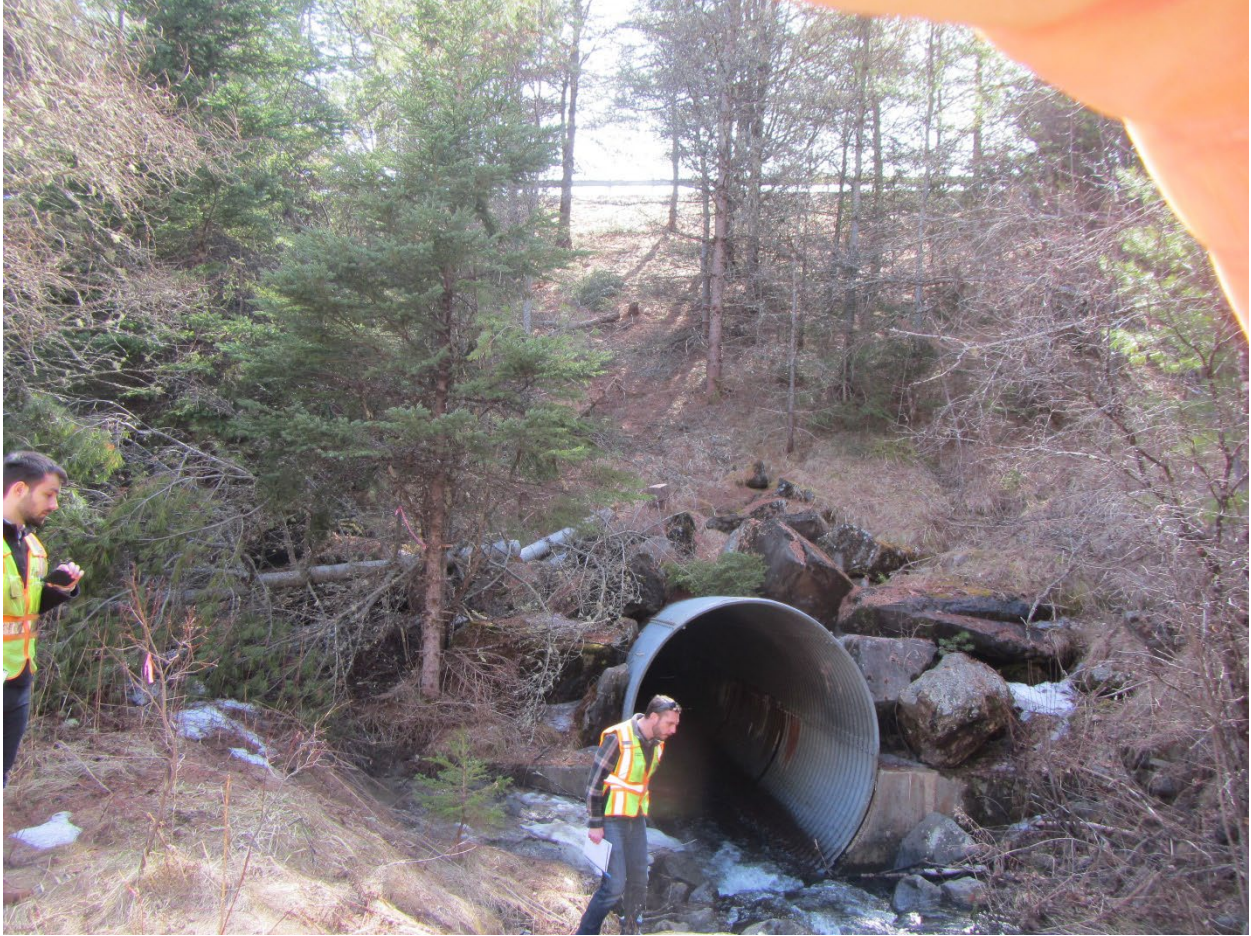
Photograph 22: Culvert 96-3S Map ID 19
