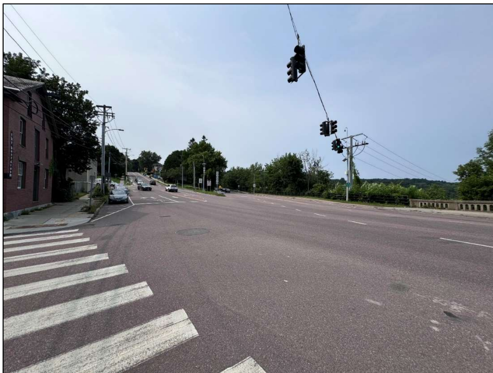
Bridge 150 Adjacent South Intersection, Looking South
