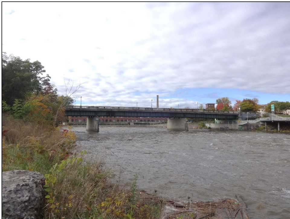
Bridge 150 Elevation, Looking West October 14, 2022
