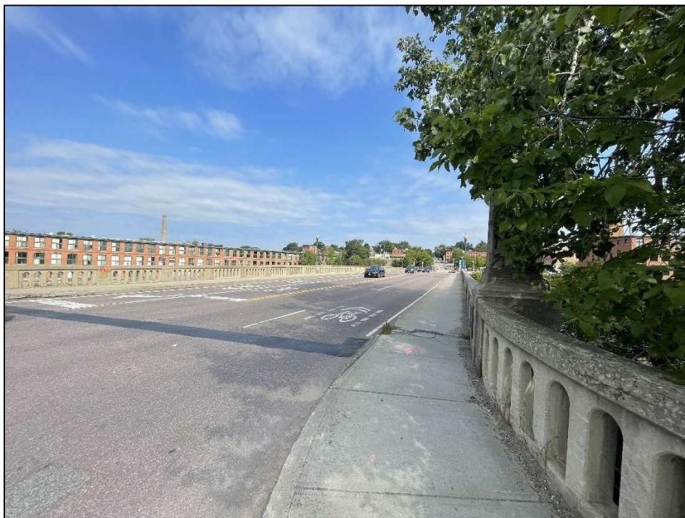
Bridge 150 Top of Deck, Looking North
