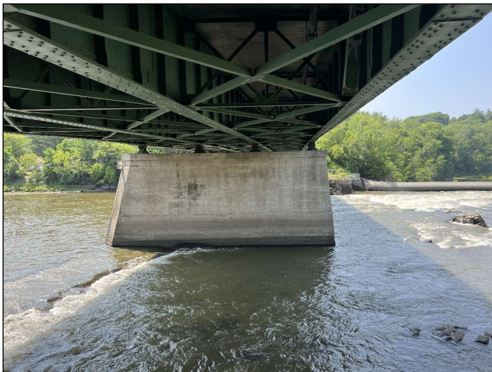
Bridge 150 Pier Elevation, Looking South
