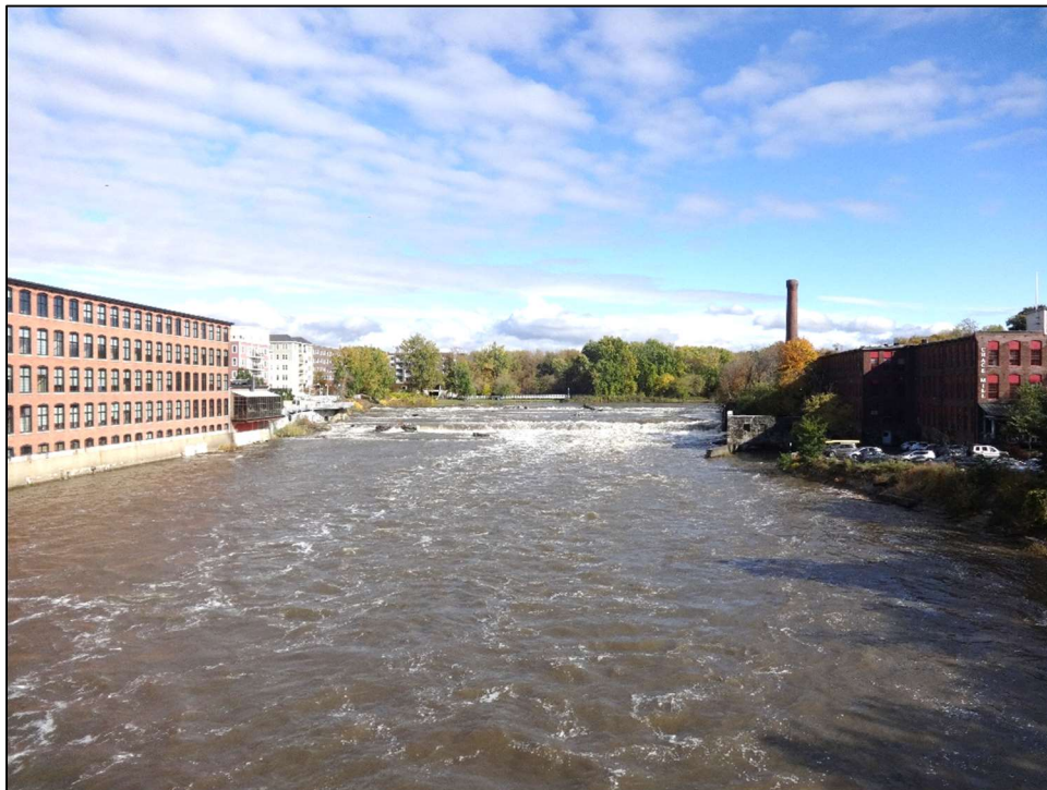
Upstream, Looking East October 14, 2022
