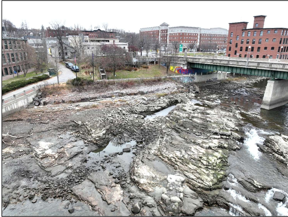
Dam Drawdown, Looking Towards Winooski Falls Park
