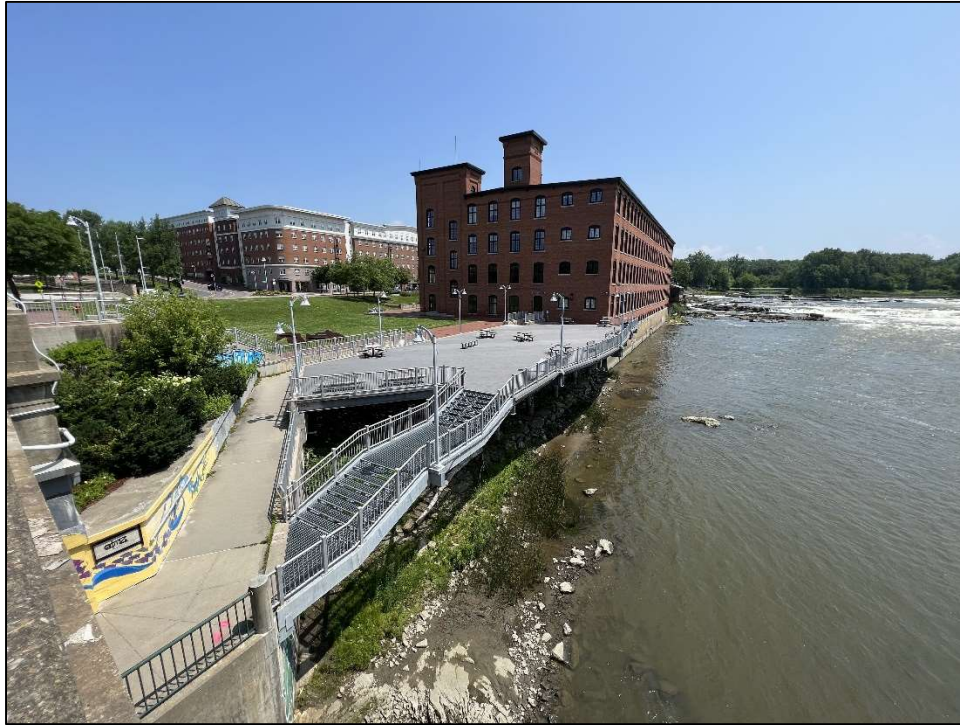
Bridge 150 Adjacent Deck and Building, Looking East
