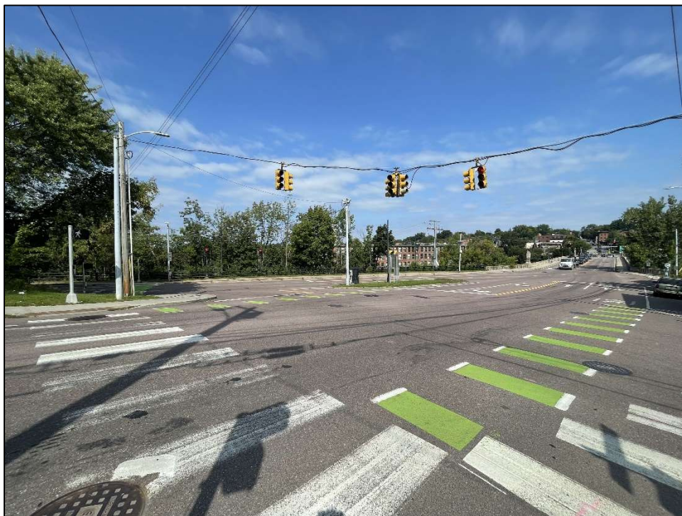
Bridge 150 Adjacent South Intersection, Looking Northwest
