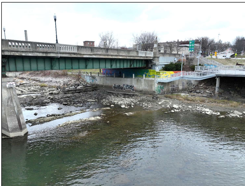
Dam Drawdown, Looking Northwest at Winooski Under-Bridge Path
