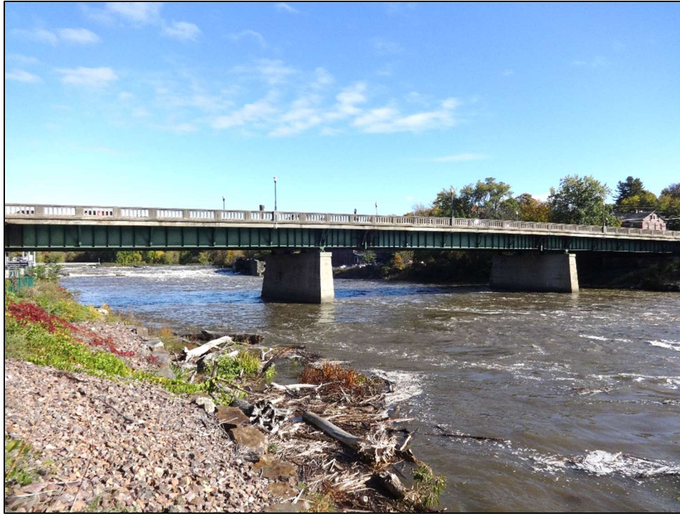
Bridge 150 Elevation, Looking East October 14, 2022
