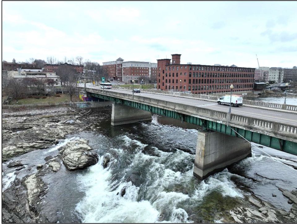
Dam Drawdown, Looking Northeast December 3, 2024
