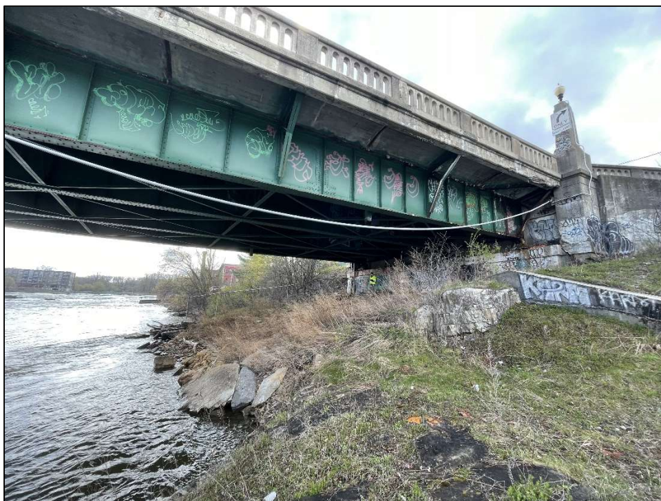
Bridge 150 Girders and Deck Overhang, Looking East
