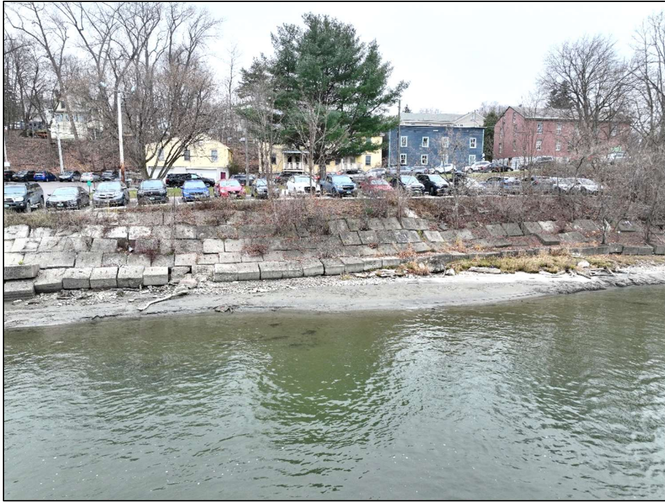
Dam Drawdown, Looking South Towards Chace Mill Parking and Mill Street
