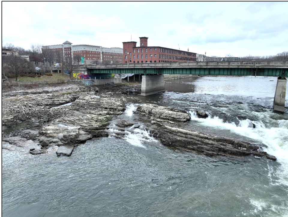
Dam Drawdown, Looking Northeast December 3, 2024
