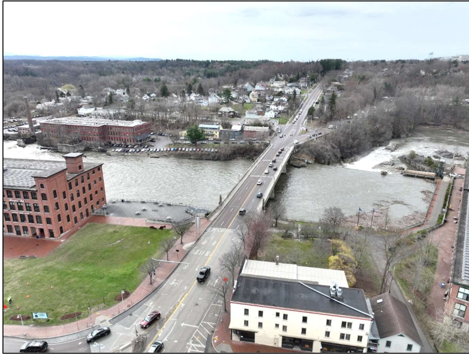
Bridge 150 General View, Looking South April 10, 2024
