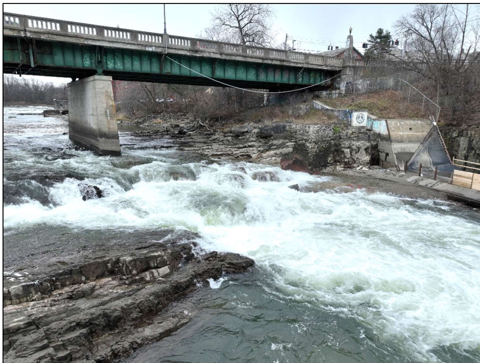
Dam Drawdown, Looking at Southwest Bridge Corner
