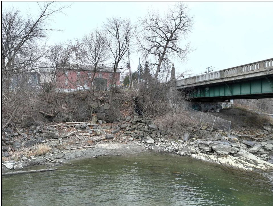
Dam Drawdown, Looking at Southeast Quadrant of the Bridge
