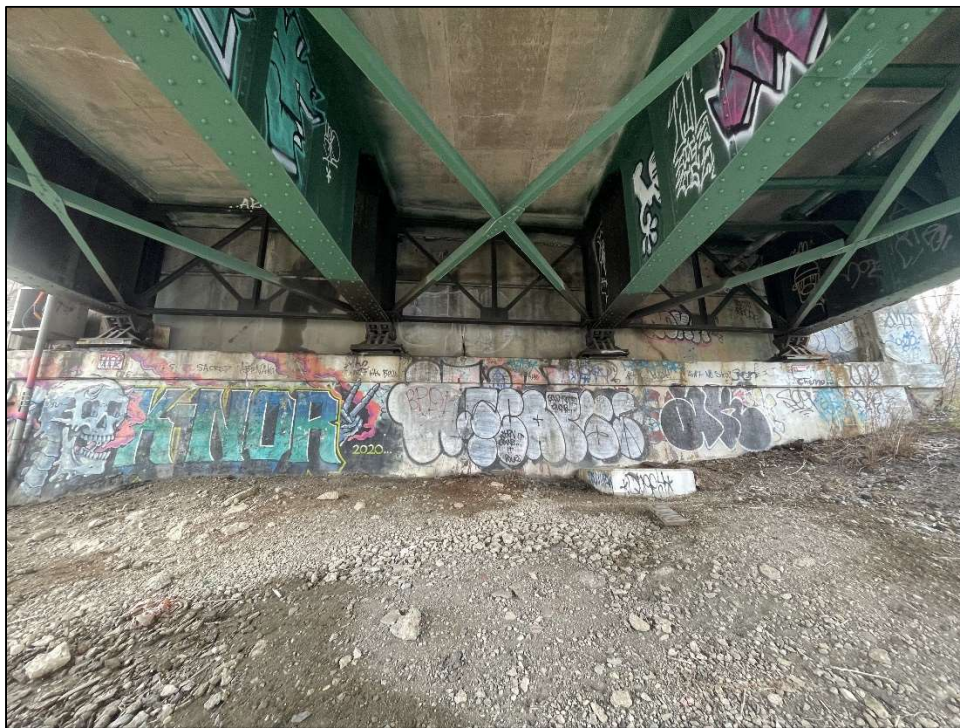
Bridge 150 South Abutment Elevation, Looking South
