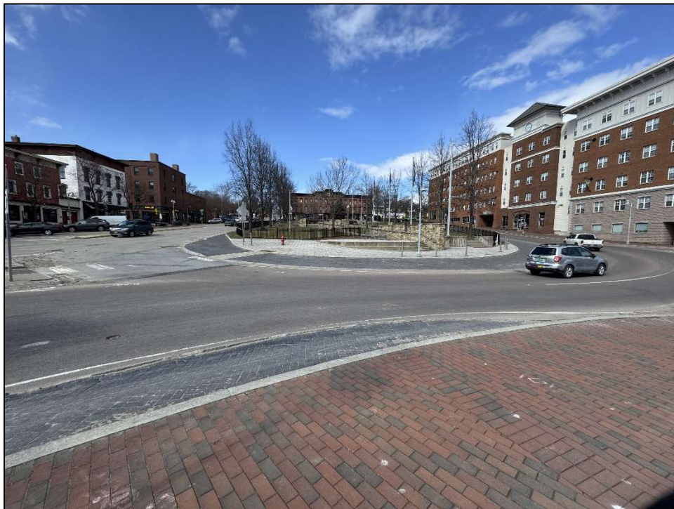
Bridge 150 Adjacent North Intersection, Looking North
