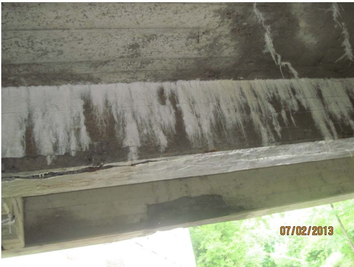
Efflorescence and crack saturation.
