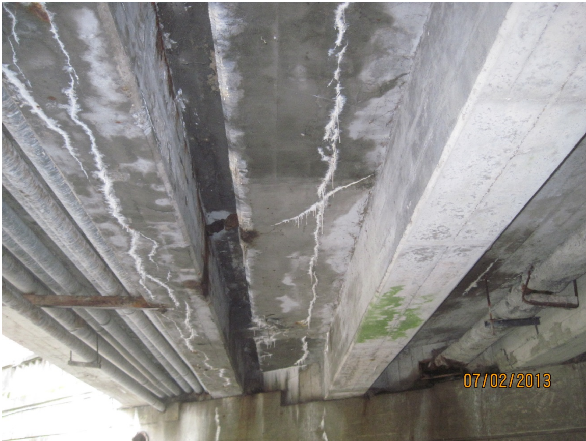
Cracking and saturation of existing T-beams.
