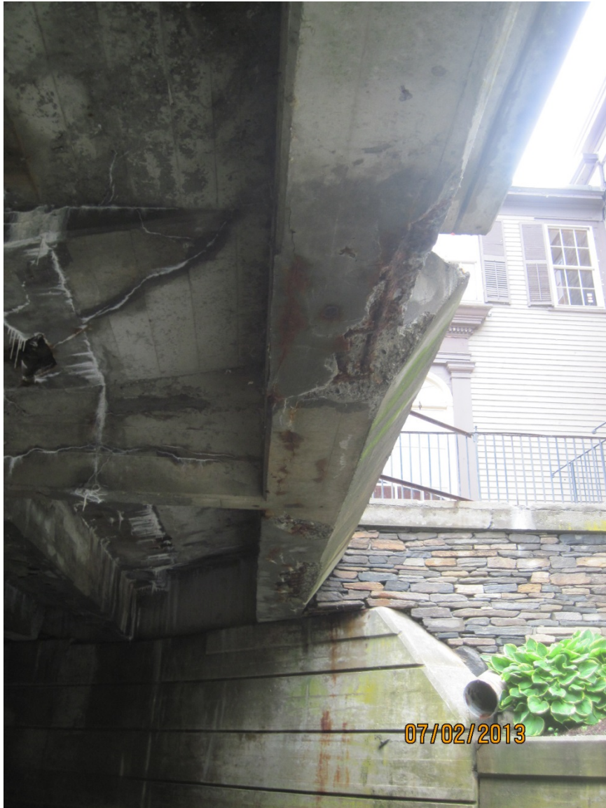
Fascia and T-beam deterioration.
