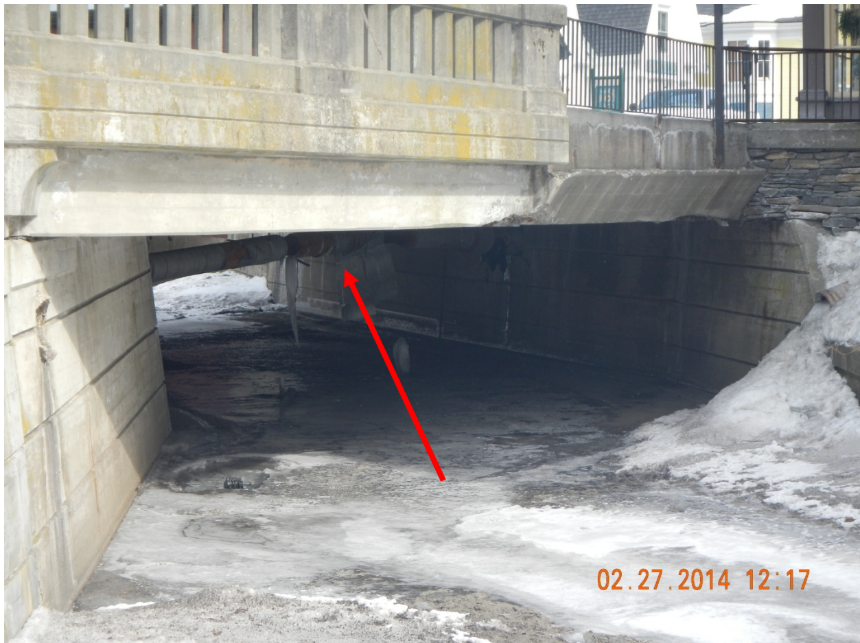
Figure 2: Electrical Conduit Running under Bridge 51
