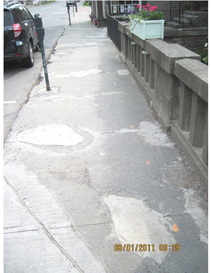
Sidewalk deterioration.
