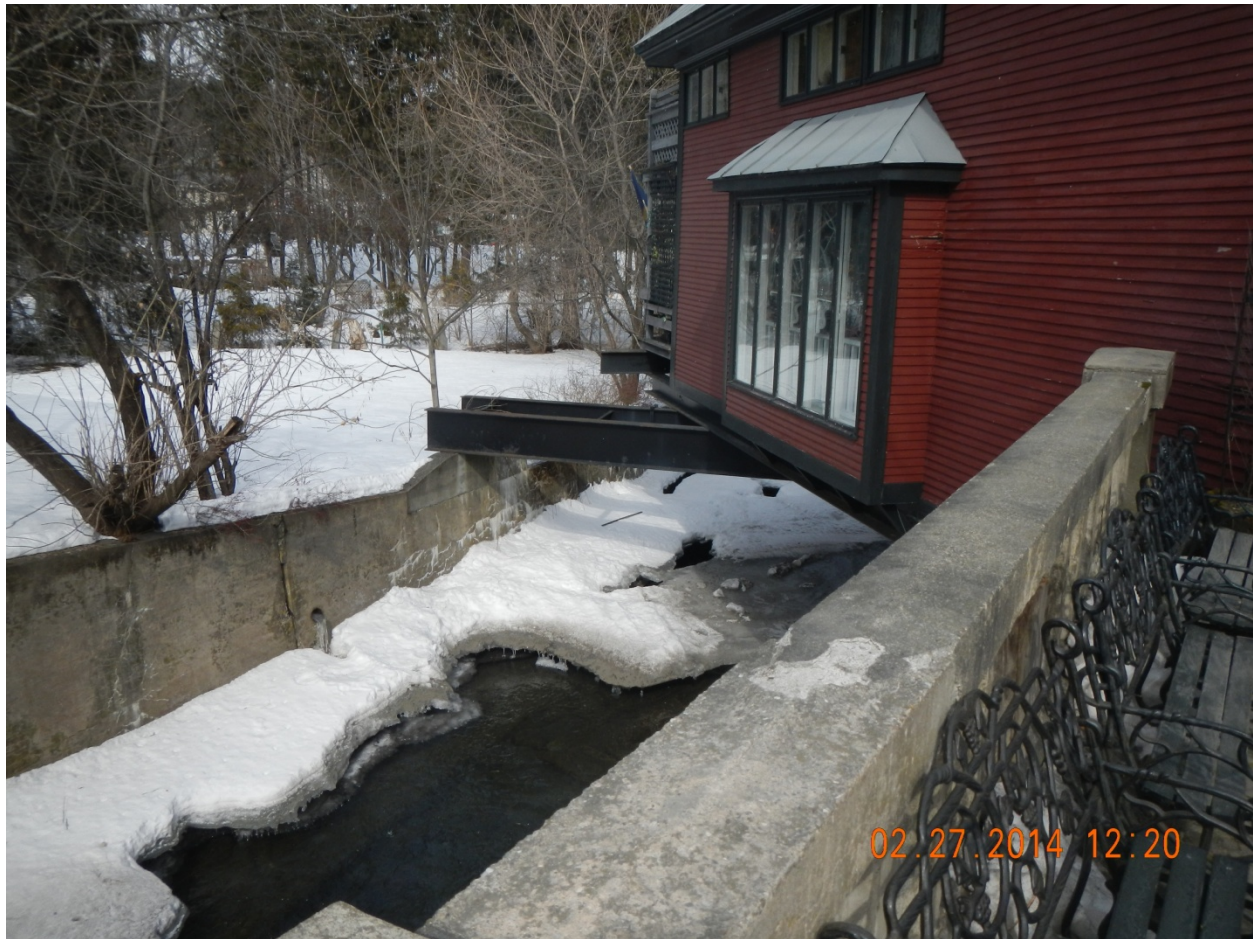
Figure 4: Building Supported on Channel Wall North of the Bridge
