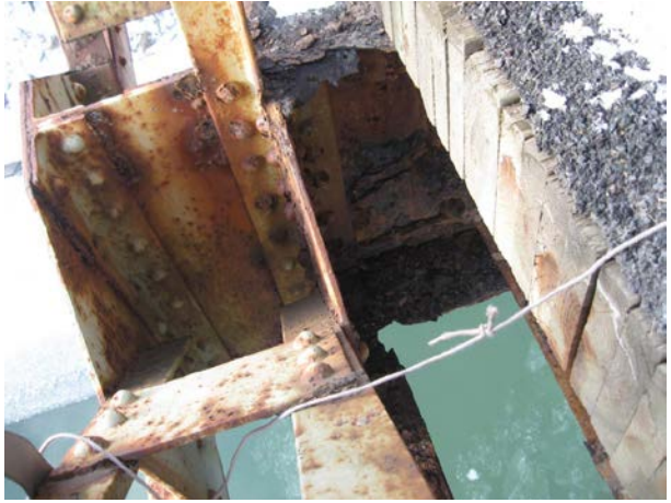
Gusset Plate distortion.
