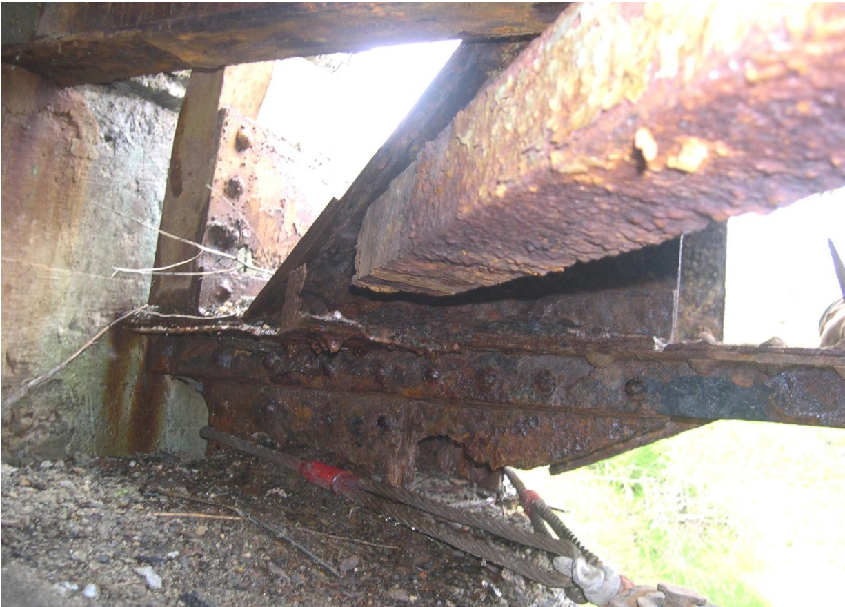
Figure 2. Truss Failure and Severe Rust Deterioration
