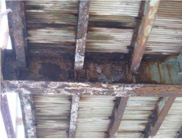
Floor beam deterioration.
