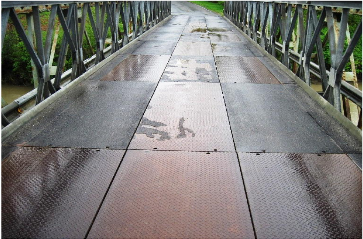
Figure 3. Temporary Bridge – Deck View
