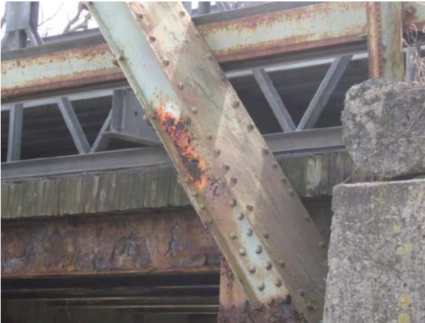
End post section loss (TYP).
