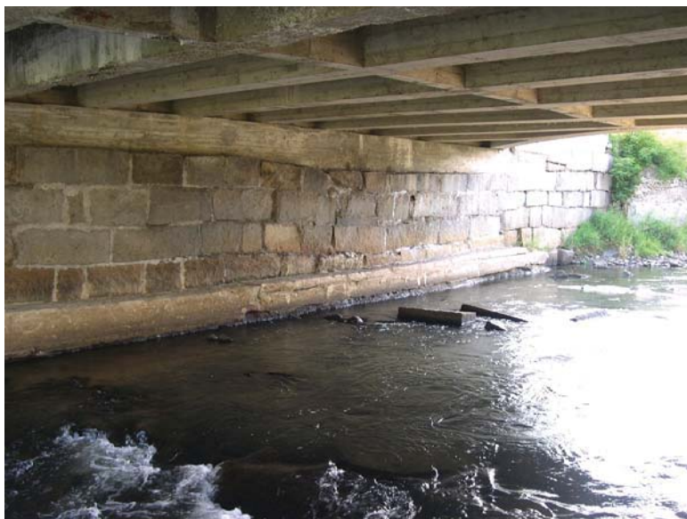
Existing Laid up Stone Abutment
