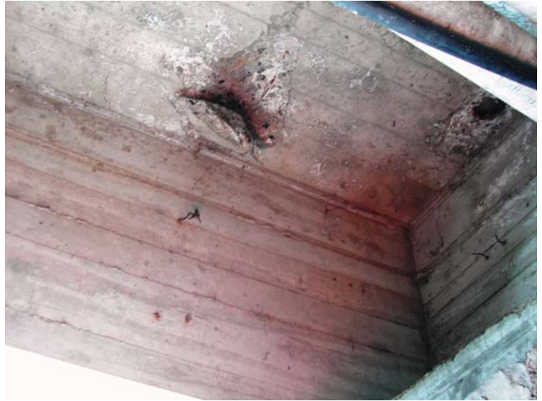
Spalling of Existing Bridge Deck
