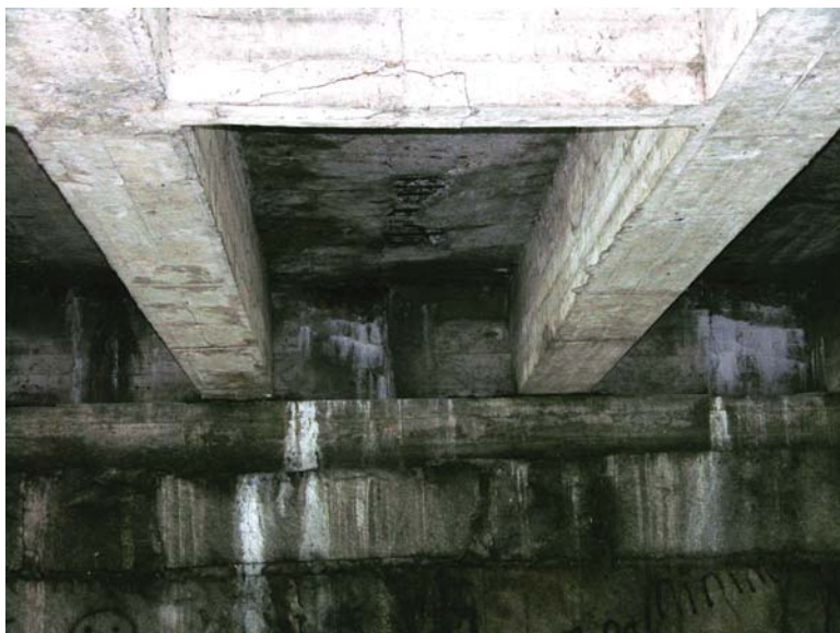
Cracking of Existing Diaphragms
