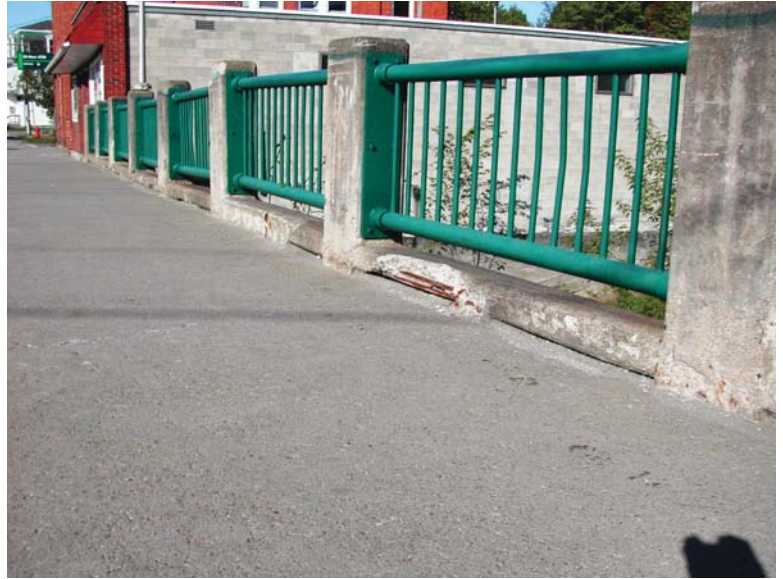
Bridge Rail Deterioration
