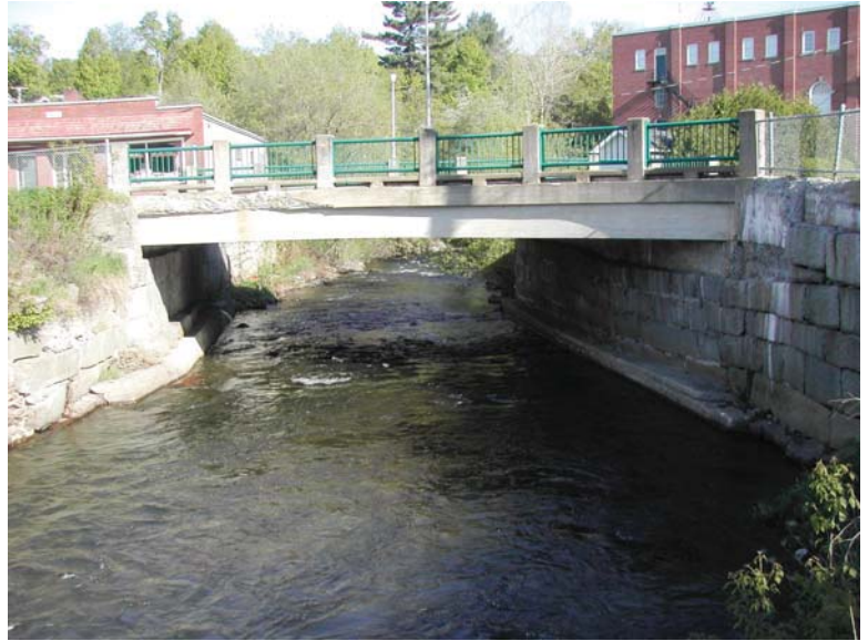
Deterioration of Southern Fascia
