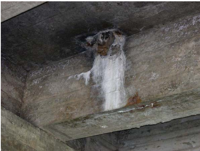
Efflorescence of Existing Bridge Deck and Beams
