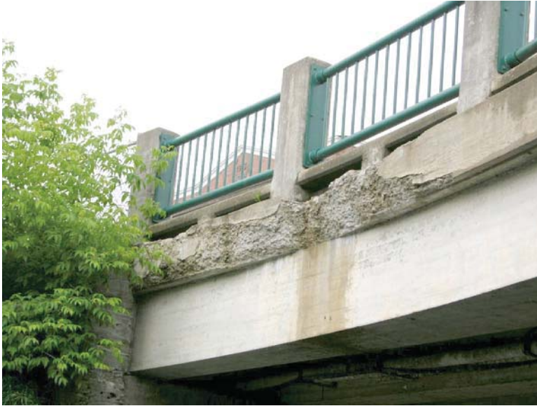
Deterioration of Southern Fascia
