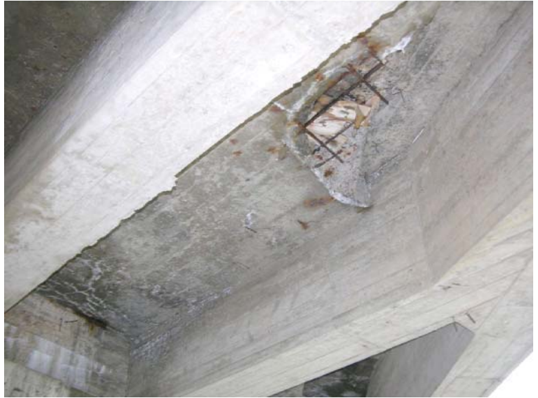
Spalling of Existing Bridge Deck
