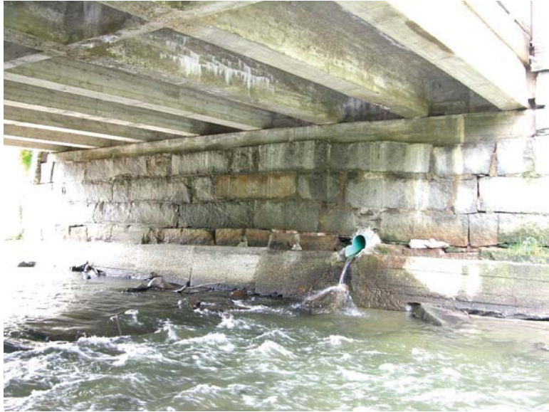
Existing Laid up Stone Abutment
