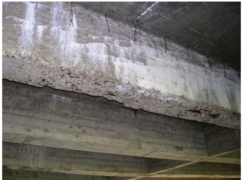
Efflorescence of Existing Bridge Beams
