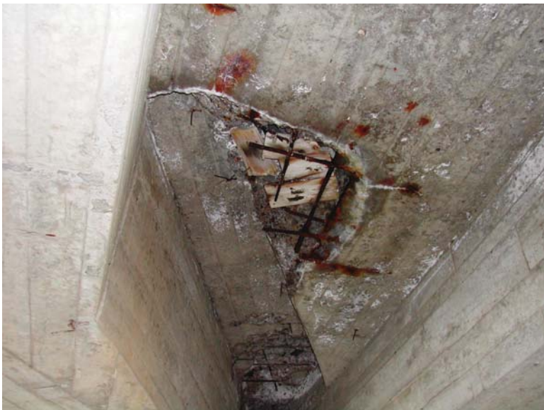
Spalling of Existing Bridge Deck
