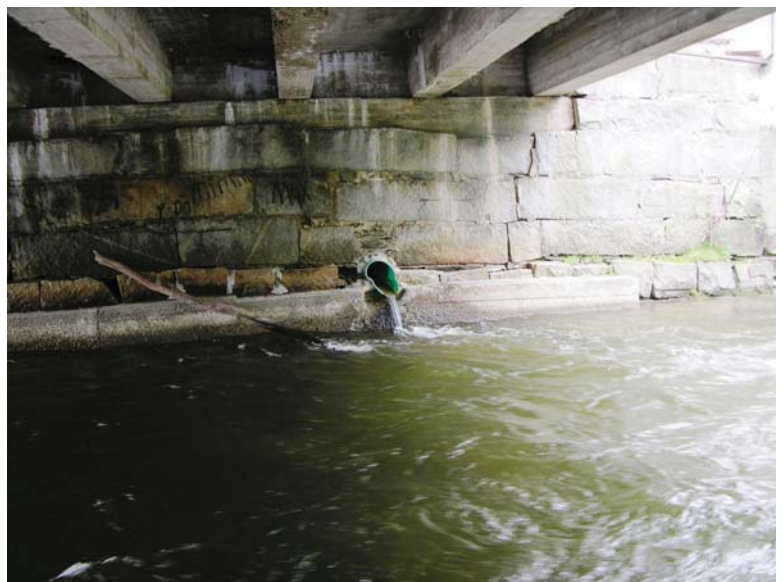
Existing Laid up Stone Abutment
