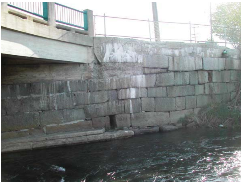
Existing Laid up Stone Abutment and Substandard Approach Rail
