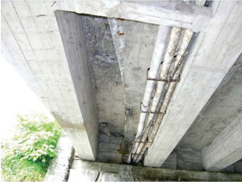
Communication Lines under Existing Bridge Deck
