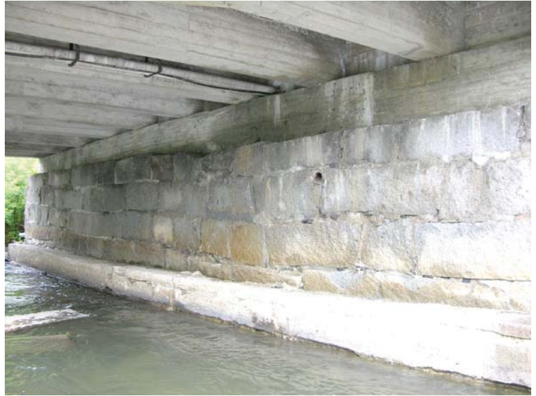
Existing Laid up Stone Abutment
