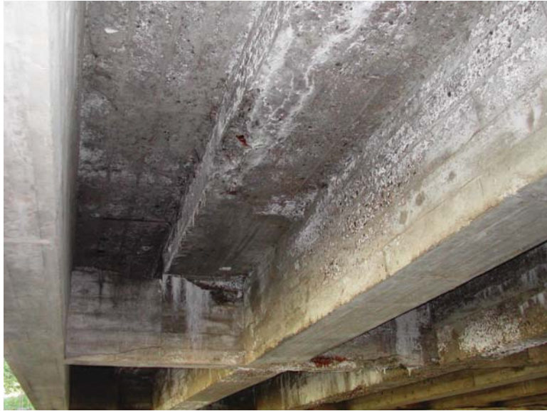
Spalling of Existing Bridge Beams
