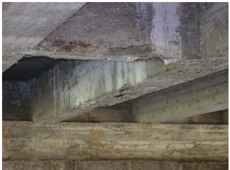
Cracking of Existing Diaphragms
