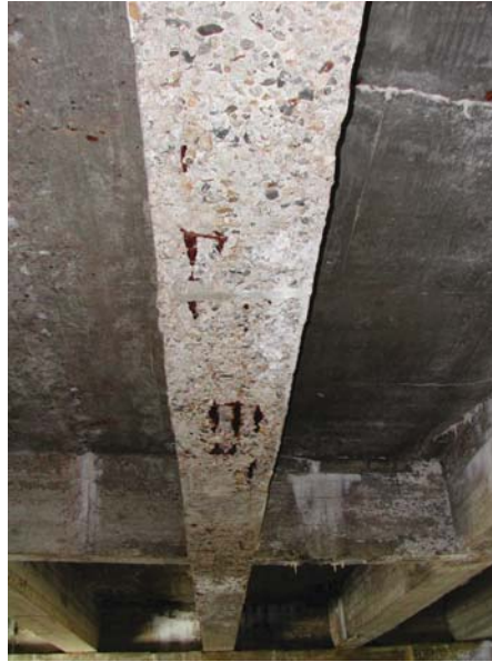
Spalling of Existing Bridge Beams
