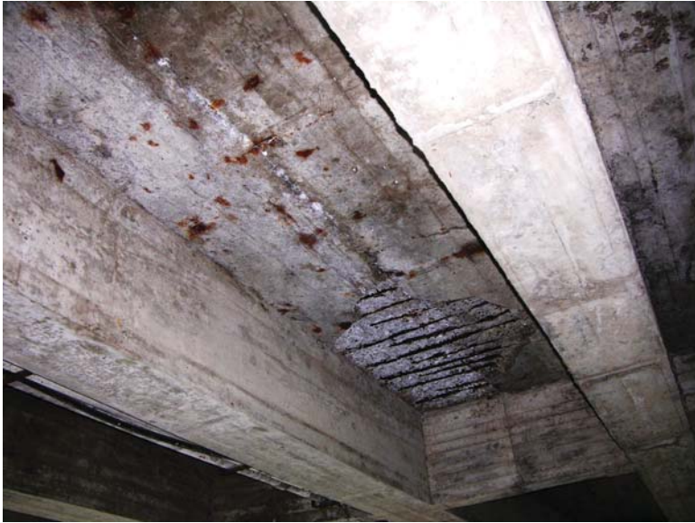
Spalling of Existing Bridge Deck
