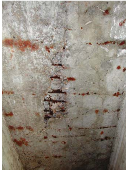
Spalling of Existing Bridge Deck
