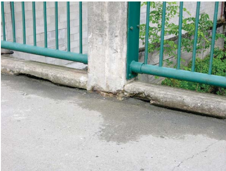
Bridge Rail Deterioration
