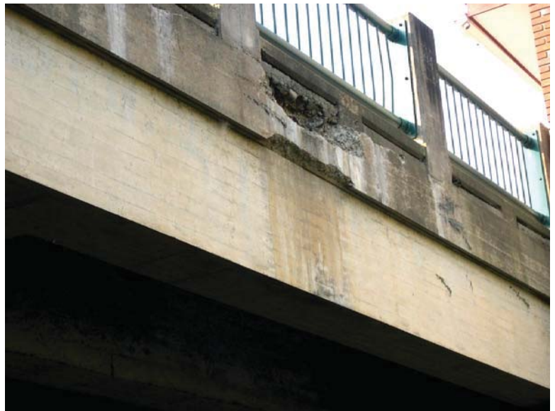
Deterioration of Northern Fascia
