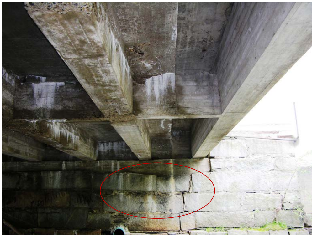
Figure 2. Broken Stone under Southern Abutment
