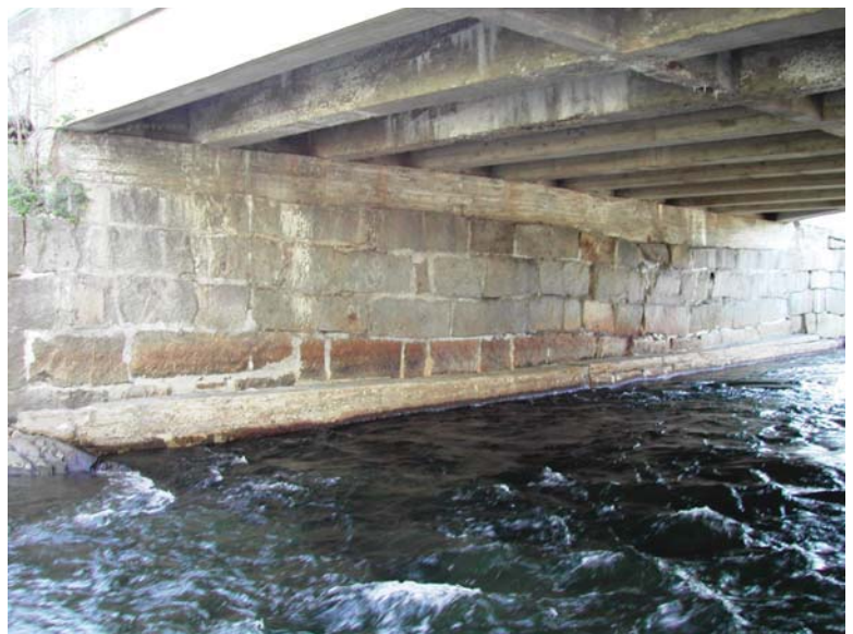
Existing Laid up Stone Abutment
