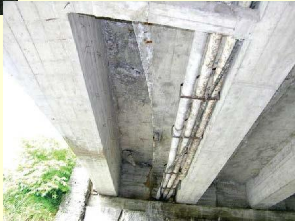
Utilities under bridge
