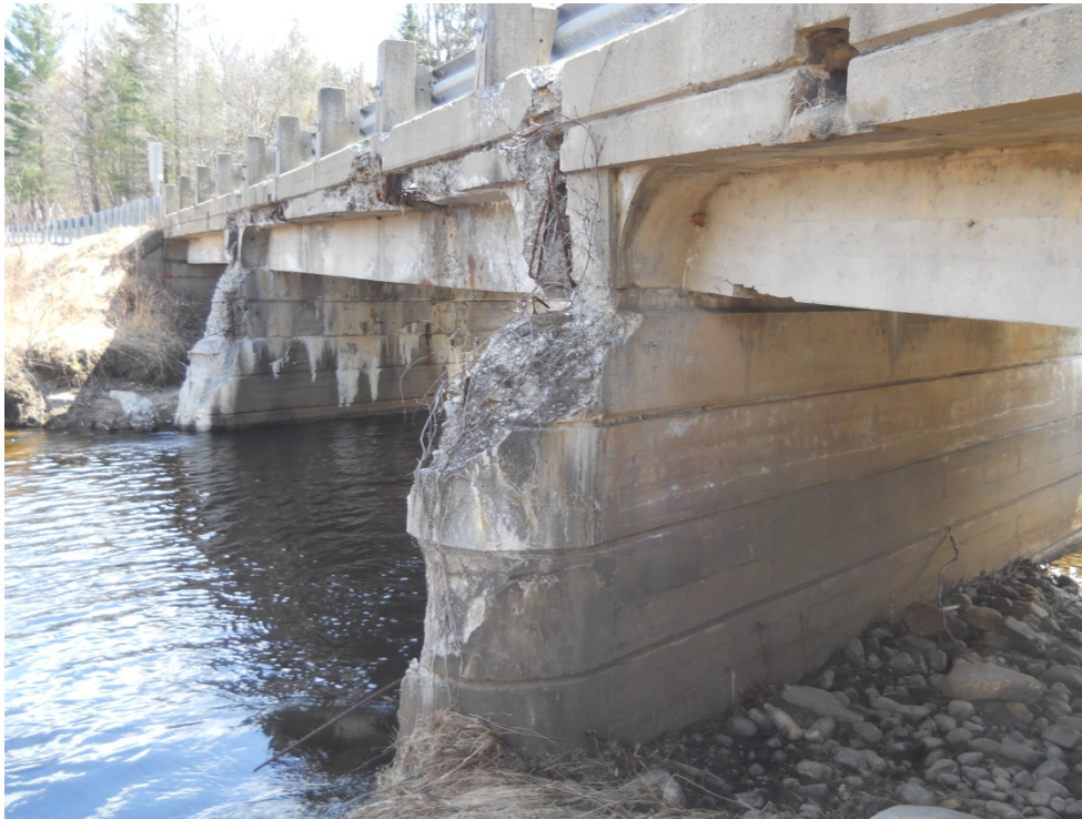
Deterioration of Fascia and Substructure
