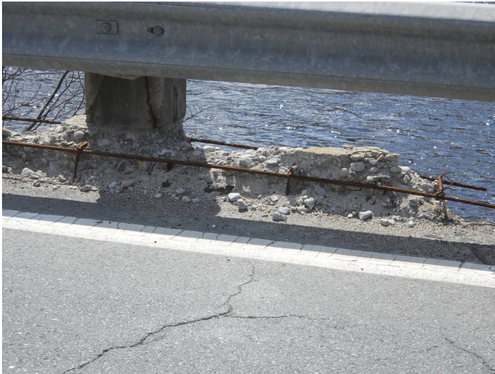
Advanced Deterioration of Curb and Fascia
