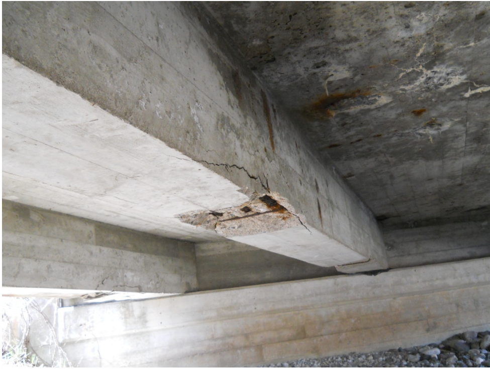
Deterioration of Tee-Beam Superstructure
