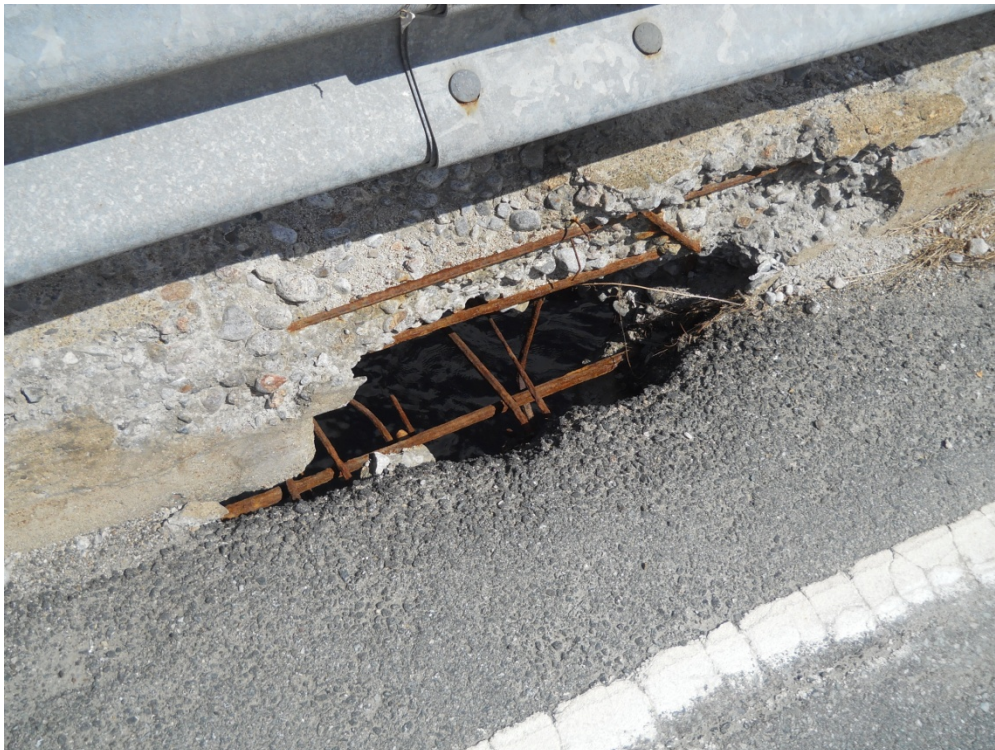
Advanced Deterioration of Curb and Deck
