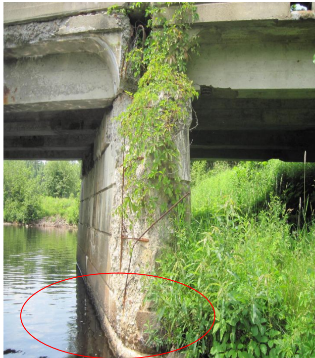
Figure 4. Undermining Developing along Pier
