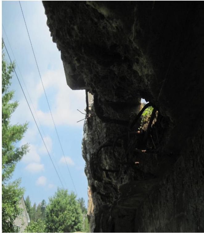
Figure 3. Severe Deck Deterioration
