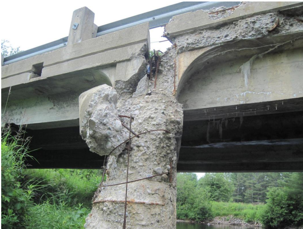
Figure 2. Severe Pier Deterioration
