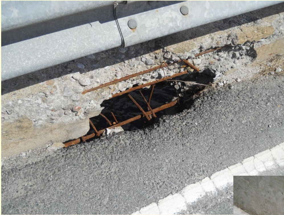
Hole in deck at curb
