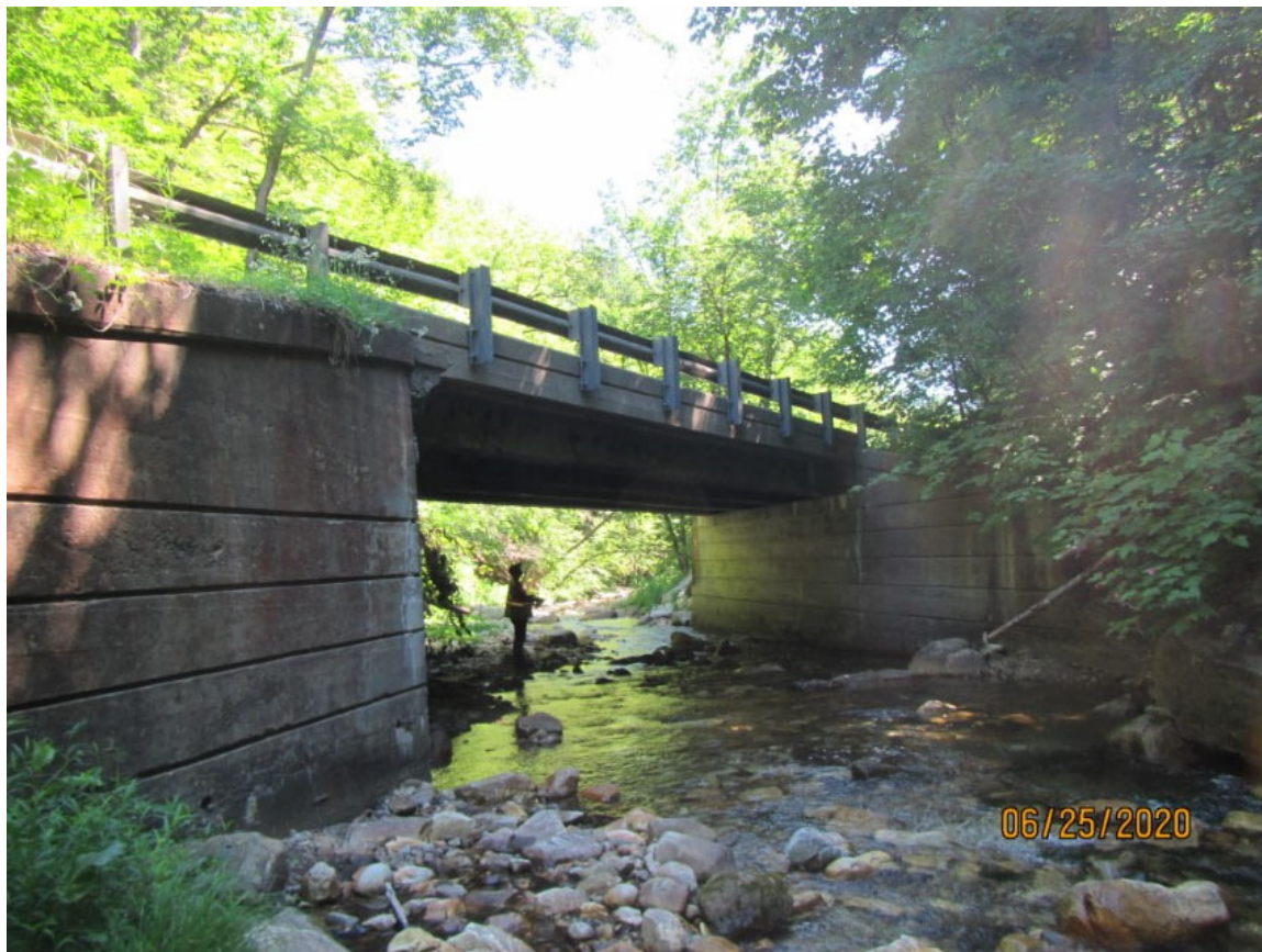
Picture 15: Upstream fascia and wingwall
