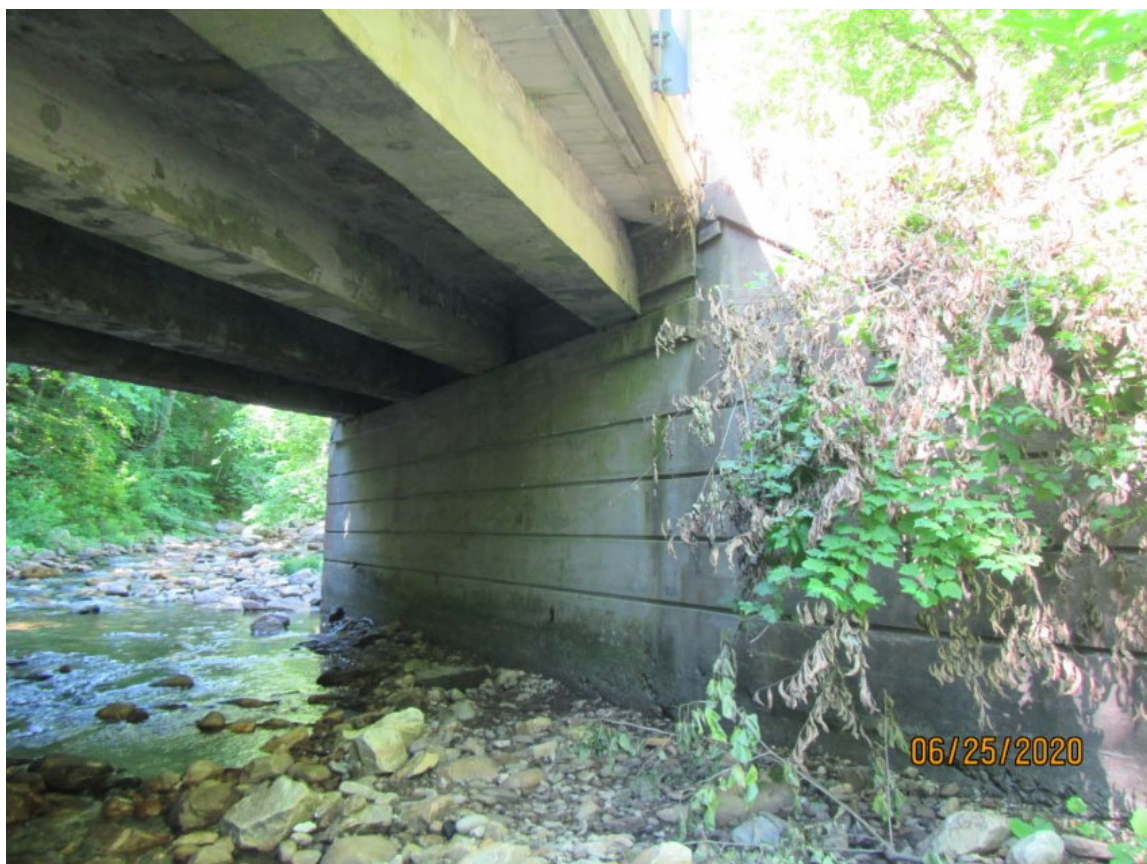
Picture 8: Western abutment
