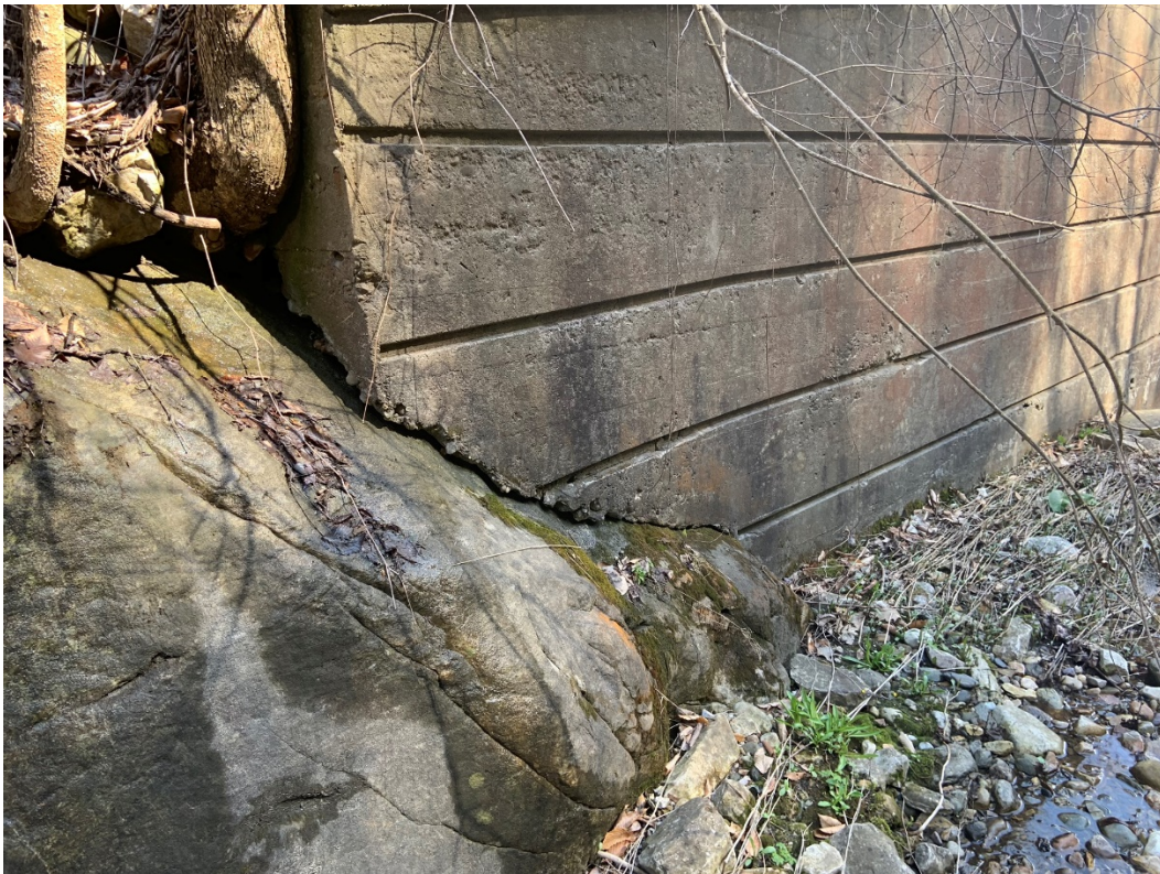
Figure 3.3: Western upstream wingwall of bridge, note wingwall cast around large boulder present.
