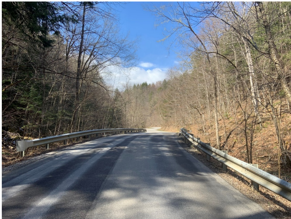
Figure 3.1: Looking west along Route FAS 0130, note no overhead utilities present near the bridge.
