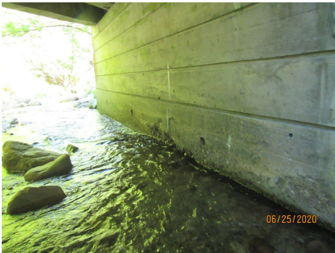
Picture 12: Eastern abutment
