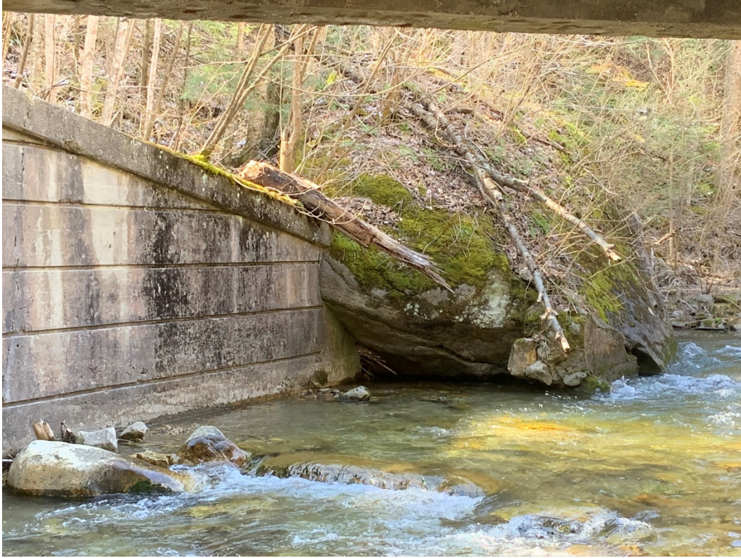
Figure 3.2: Facing eastern upstream wingwall, note wingwall cast around large boulder present.
