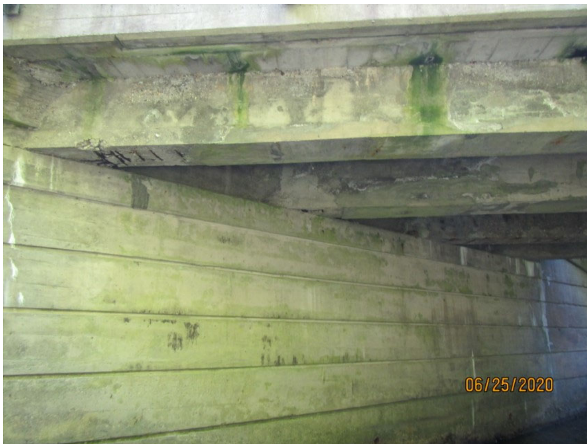
Picture 6: Eastern abutment
