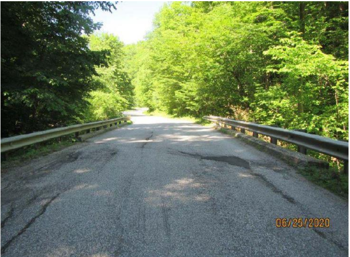
Figure 6: View of Bridge Deck.
