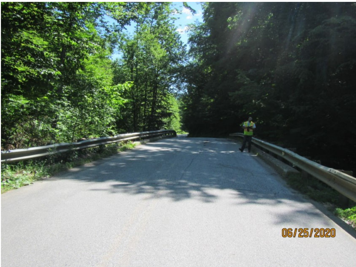
Picture 2: Looking west over Bridge 7
