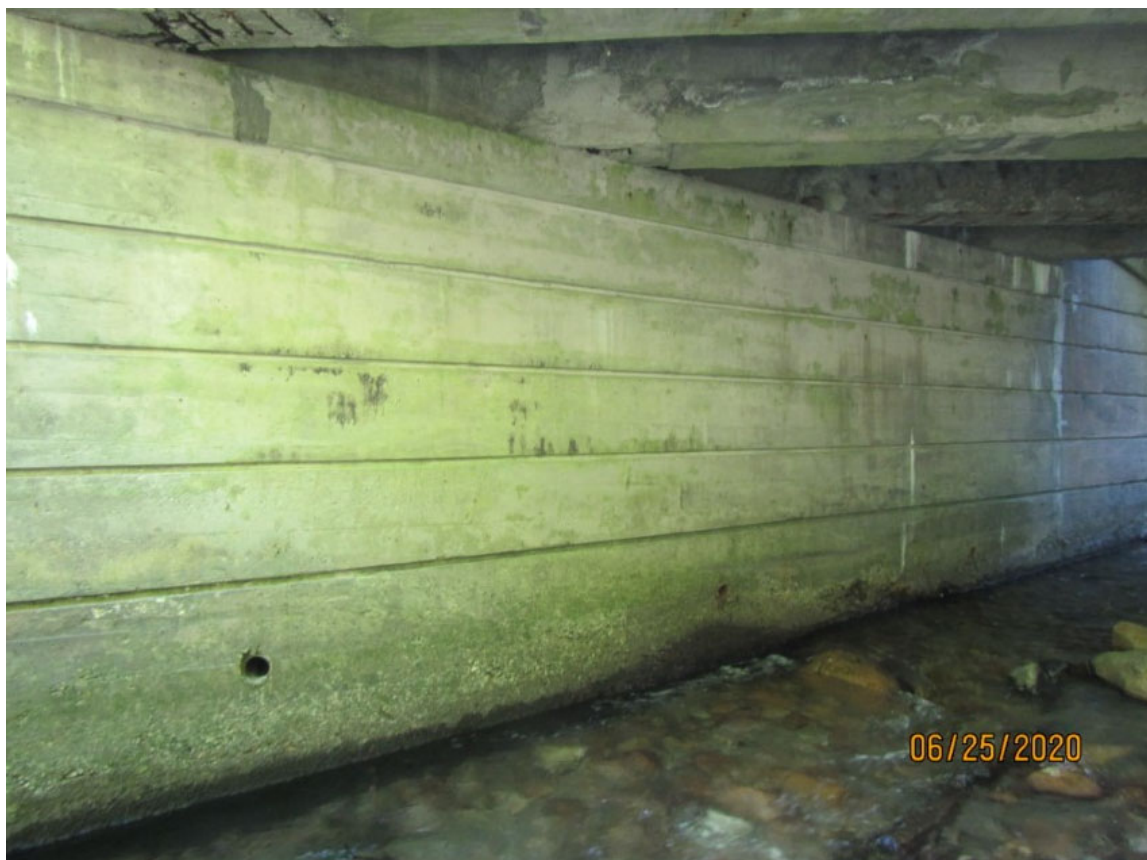
Picture 7: Eastern abutment
