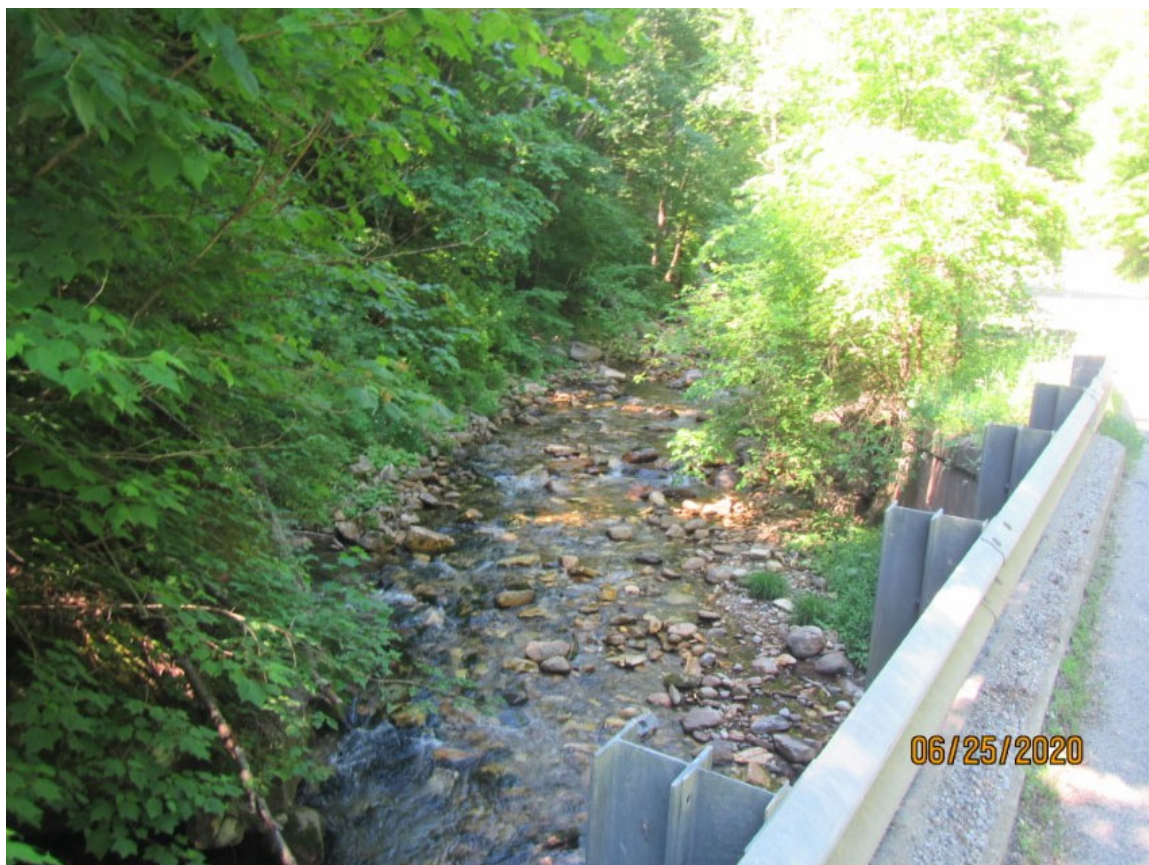
Picture 3: Looking downstream
