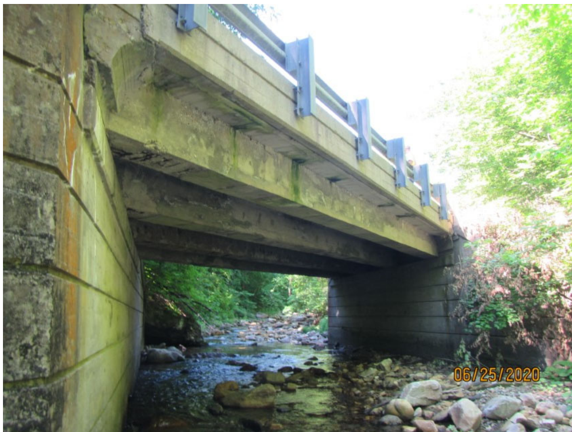
Picture 5: Downstream fascia
