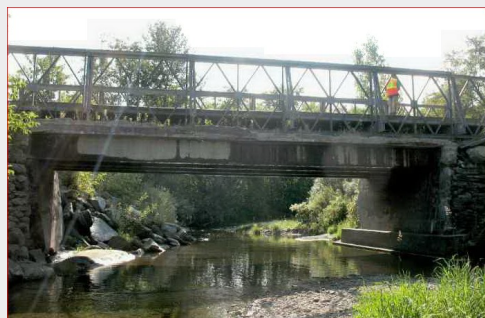
Existing abutments and steel looking upstream
