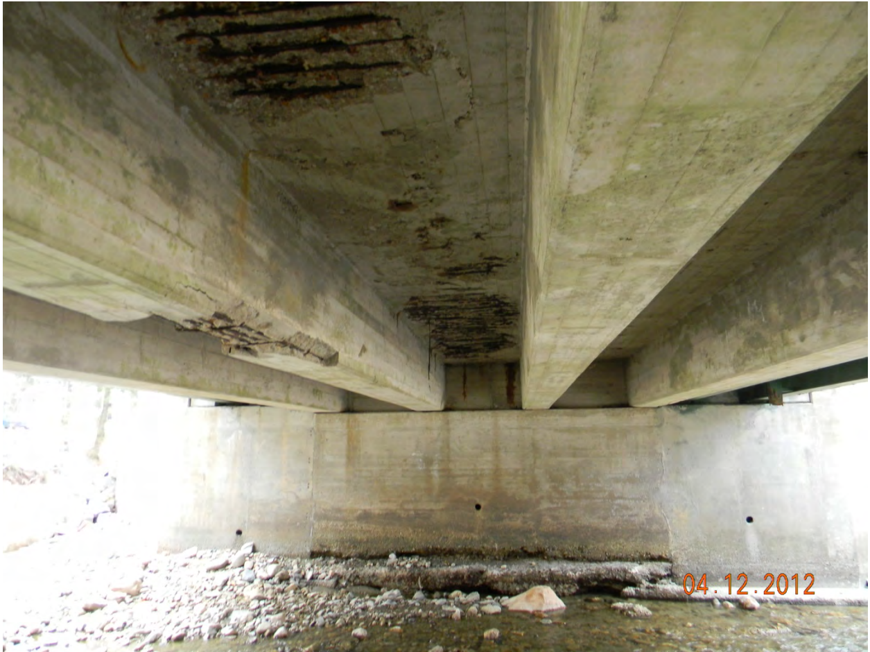
West Abutment (Note Deck/T-Beam Deterioration)
