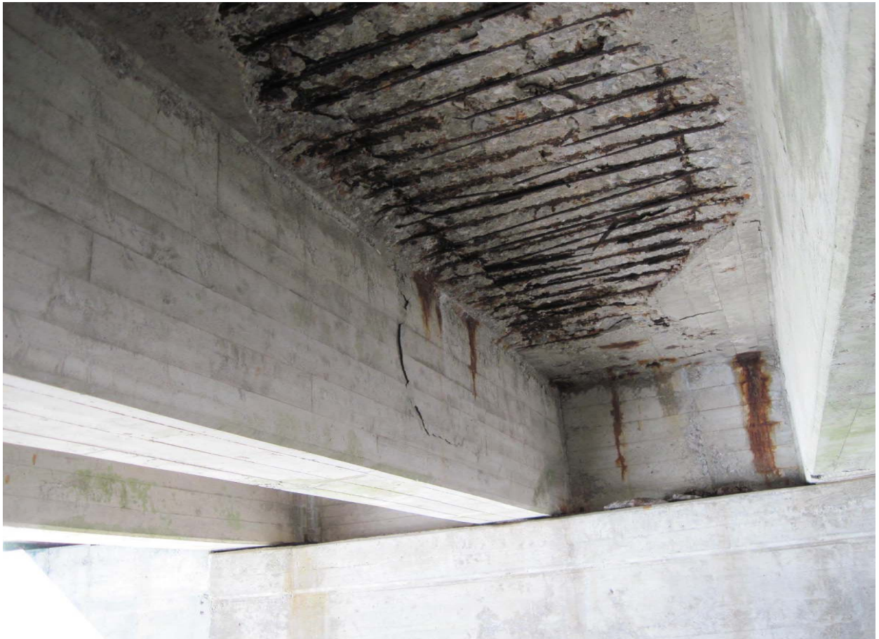
Exposed Reinforcing Steel in Deck
