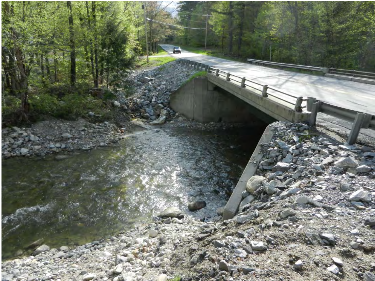
Figure 2. View of bridge, facing west.
