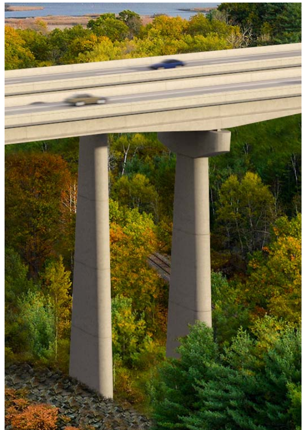
The R&R Team has Determined that a Spliced Girder Bridge Poses Significantly Less Construction and Schedule Risk Than the BTC
