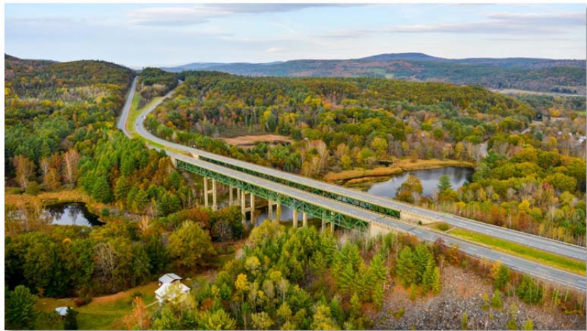
R&R's Repair Plan Implementation for the Existing Bridges Will Minimize In-Service Repairs During Construction
