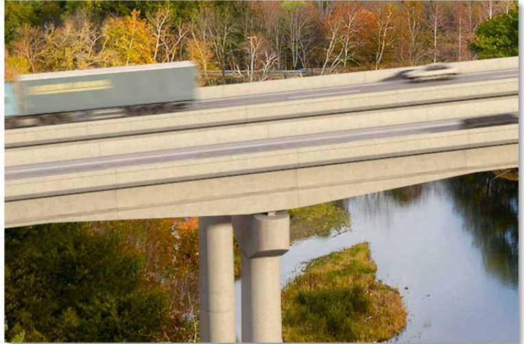
The R&R's Team's Approved ATC is a Spliced Post-Tensioned Precast Concrete Girder Structure
