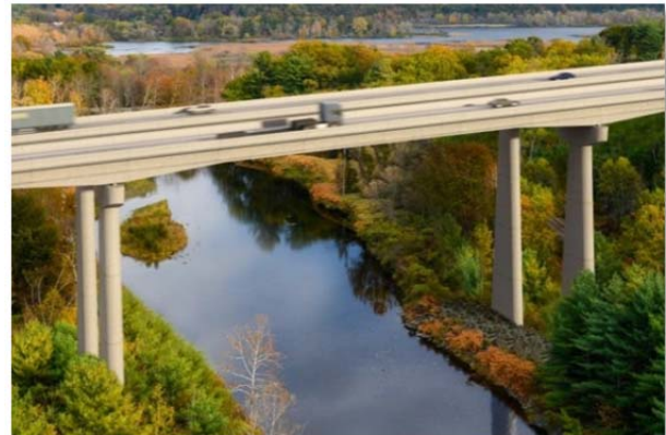
Proposed Piers are Located Behind the Existing Piers Reducing Potential Scour Impacts
