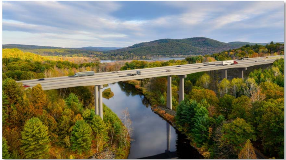
The R&R's Team's Spliced, Post-Tensioned, Precast Girder Concept will Exceed VTrans Requirement for 100-Year Service Life
