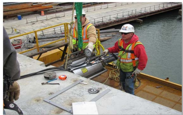
R&R Erectors have Post-Tensioning Certifications to Perform the Spliced Girder PT
