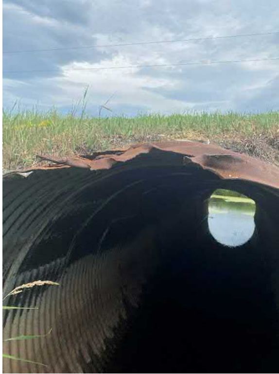
Photo 5: Culvert Outlet Corrosion Dated: 06/29/2021
