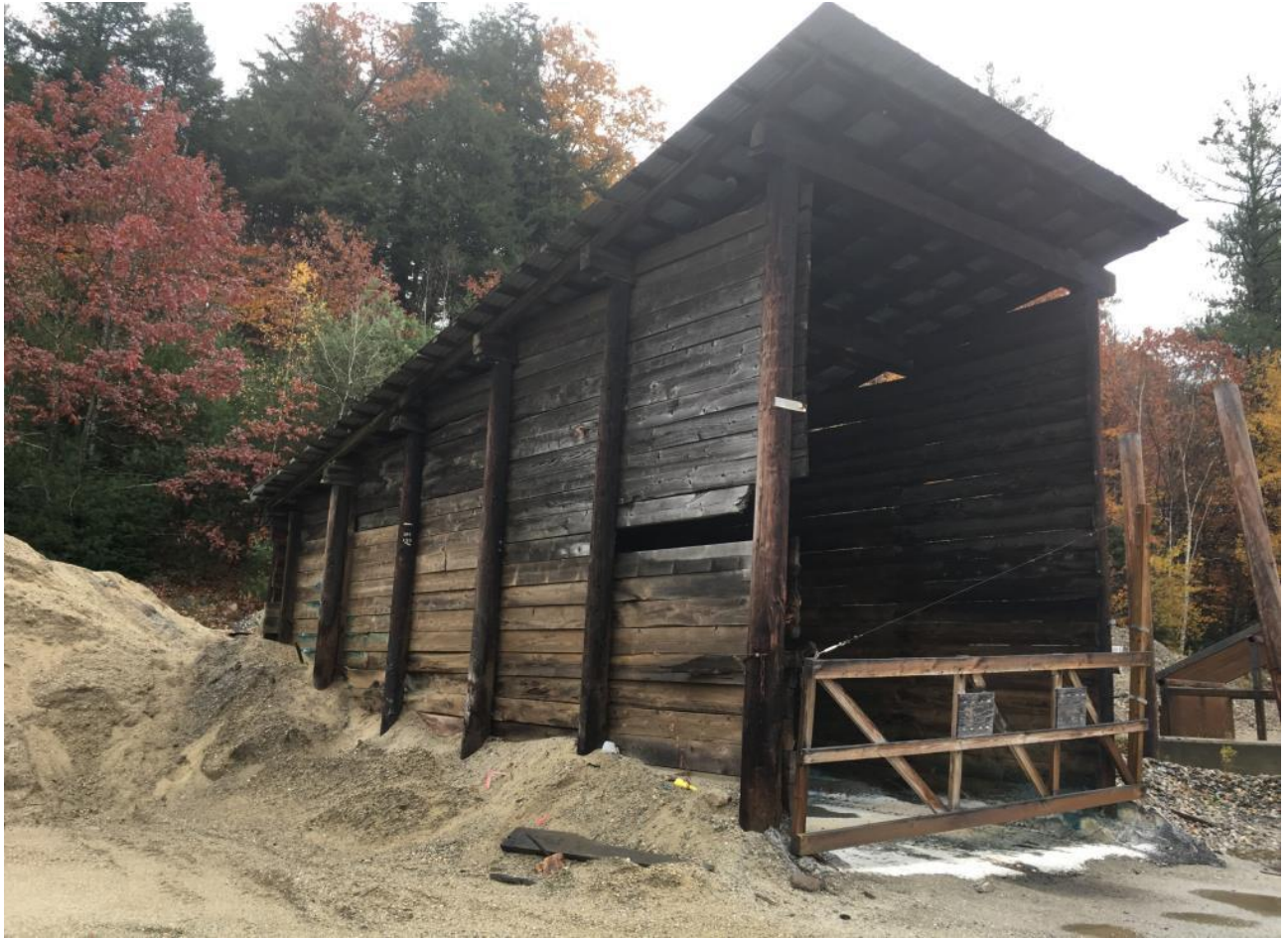
Pictures - Condition of Shed
