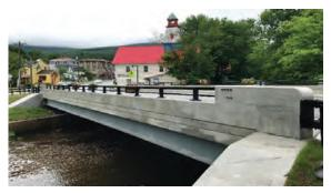
course, 8" water main replacement on structure, drop inlet structures, granite curb, black bridge rail, signage, striping, conduit and lighting and approach improvements. The new bridge features a Tenney Railing with partial height concrete parapet and steel tubing to be consistent with the adjacent Ludlow Historic Village District. WSP provided precast concrete inspection, construction inspection and office engineering.
