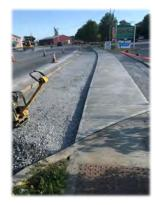
Our firm was selected by the City of Vergennes using the VTrans "At-The-Ready" roster program to provide Resident Engineering services for the Vergennes STP BP15(6) Pedestrian Improvements Project. The project included new 5' wide concrete sidewalks, stormwater improvements, and new Rapid Rectangular Flashing Beacon
