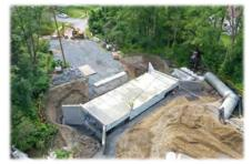
Our firm provided Resident Engineering, Construction Inspection, and Testing Services for the replacement of two deteriorated 6-ft diameter x 70-
