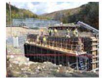
removed and a new abutment and 1-span of a 3-span steel girder bridge was constructed.
