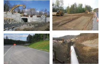
**Town of Sharon FEMA Repair to Route 132 and River Rd., VT.** Construction engineering & testing Inspection services, which involved traffic plan layout, removal of pavement at damaged locations, repair of guardrail, installation of new guardrail, roadway shoulder repairs, grass and stone swale repairs, pavement markings and removal of sediment debris.
