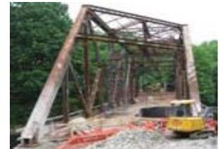
**Springfield BHO 1442(30), VT.** Provided construction inspection of rehabilitation of existing truss along with related substructure and channel work.
