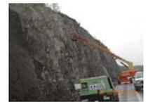
**Berlin-Montpelier IM 089-1(53), VT.** Included hand rock scaling, rockfall catchment fence installation, traffic control and related work. Assisted resident engineer in overseeing removal of ledge by hand scaling, installation of rockfall fence, and the removal and resetting of guardrail. Assured contractor complied with the erosion control plan and completed work in a safe manner.
